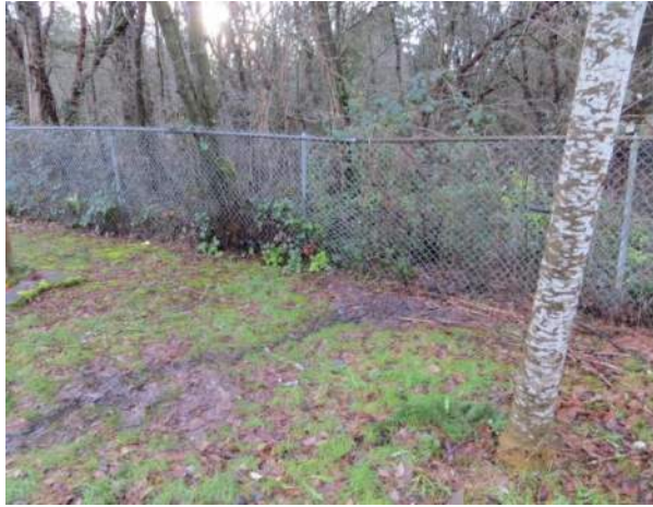
Photo 4. Runoff from the parking lot currently flows under the fence and downhill to the park property to the south.
