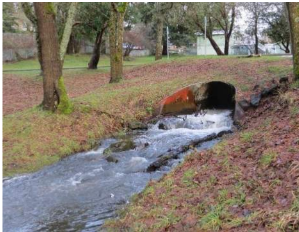
Photo 12. Stream flowing out of culvert south of park drive.
