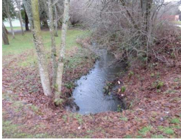
Photo 11. Stream just north of park drive entering culvert under driveway.
