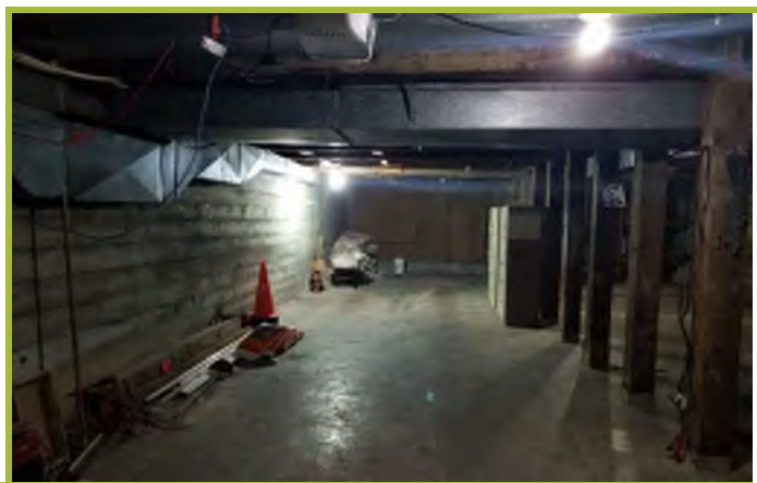
Photograph #20: Garage (unused) – basement level.
