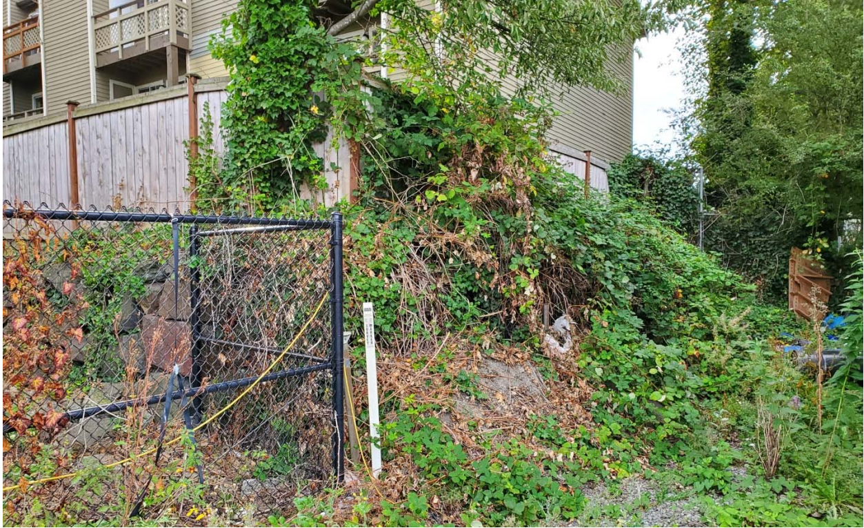
Photo 3: Rockery along eastern perimeter of site, looking southeast.
