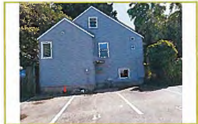
Photograph #42: Manager's residence for multi-family development south of 10724 Avenue SW. Looking south.
