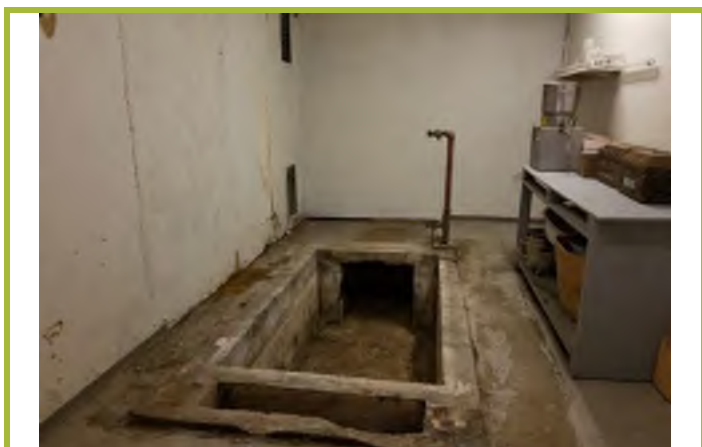
Photograph #17 Abandoned crematorium (1) – basement level.
