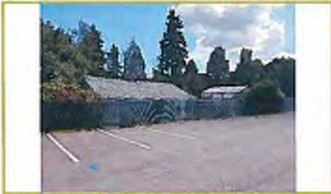
Photograph #37: View from Yarrington's Funeral Home parking lot looking southeast toward adjoining property at 1511 SW 107 th Street.
