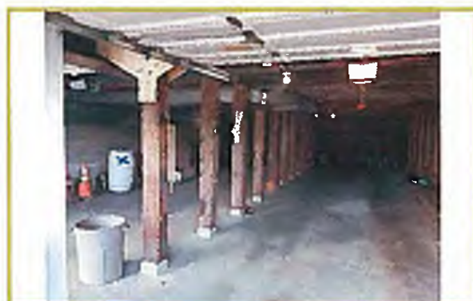
Photograph #17: Garage entrance in basement.
