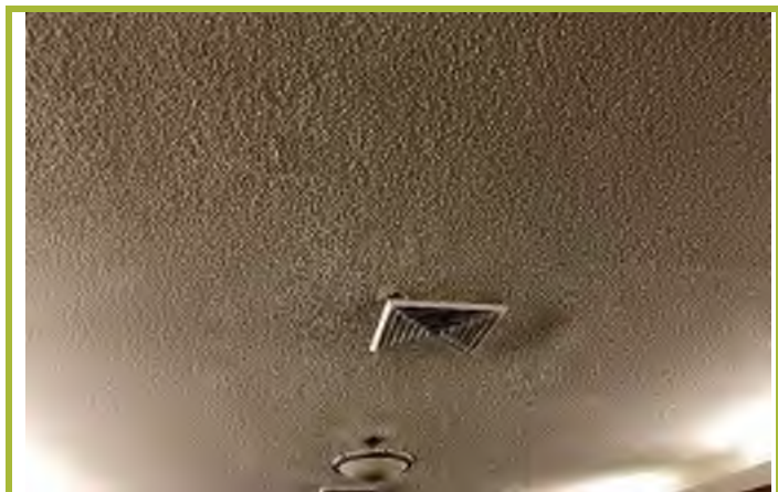
Photograph #12: Typical 'popcorn' ceiling on funeral home main floor.
