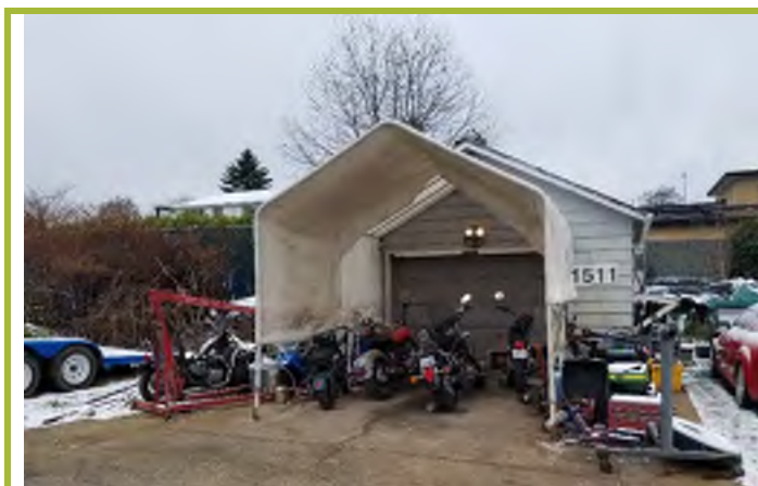
Photograph #6: Exterior view of single car garage associated with the Huddleson residence (2 of 2). Looking west.
