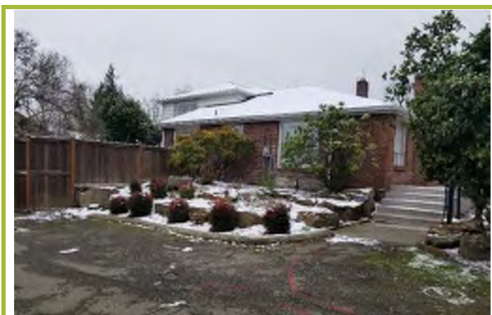
Photograph #5: Manager's residence for Yarington's Funeral Home (10724 16 th Avenue SW). Looking southeast from funeral home.
