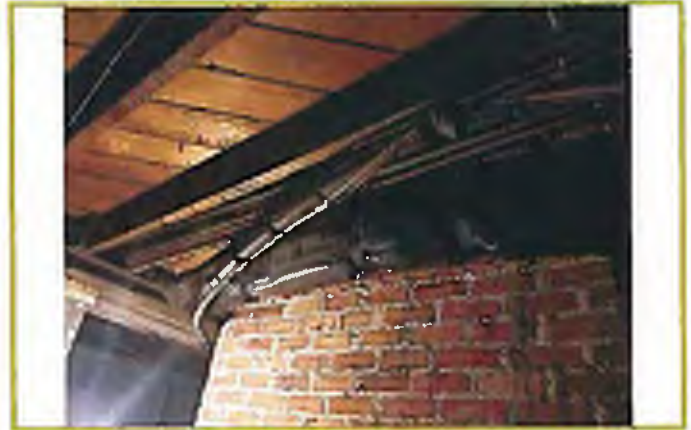
Photograph #20: View from basement, showing typical construction and materials.
