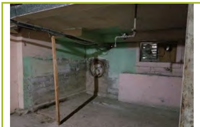
Photograph #18: Abandoned crematorium (2) - basement level.
