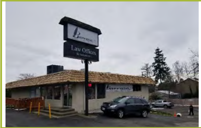
Photograph #37: Barraza Law Office, located south of funeral home manager's residence. Looking northwest from 16 th Avenue SW.
