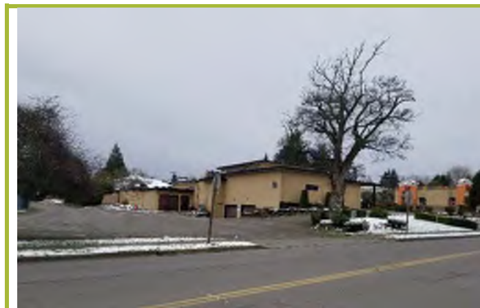
Photograph #4: Rear view of Yarington's Funeral Home from SW 107 th Street. Looking southeast.
