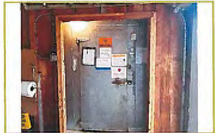
Photograph #22: Door for cadaver storage freezer - basement level.
