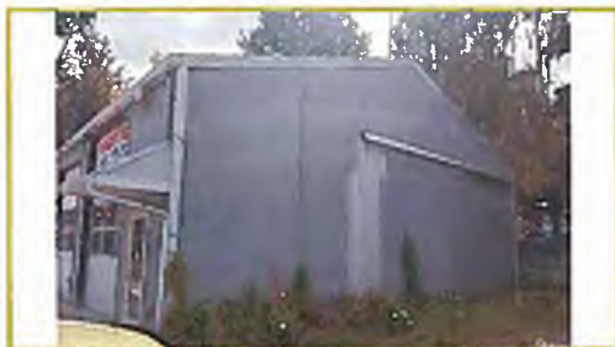
Photograph #9: Second view of RWT Window Tinting shop building exterior. Looking east-southeast.
