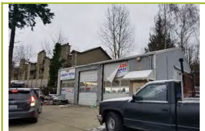
Photograph #4: RWT Window Tinting shop building exterior. Looking southeast.
