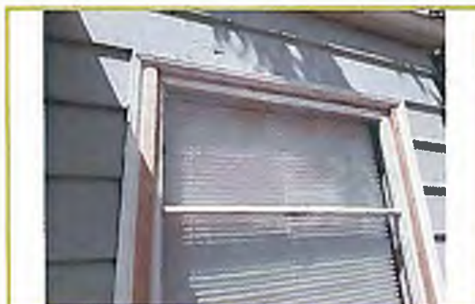
Photograph #5: Detail of exterior building materials, Huddleson property residence.
