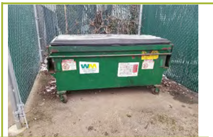
Photograph #28: Waste Management garbage dumpster – rear parking lot.
