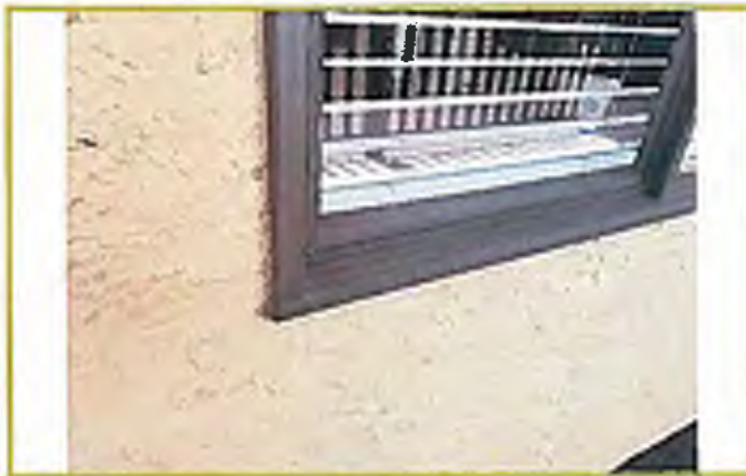
Photograph #27: Detail of typical building materials facing 16 th Avenue SW.
