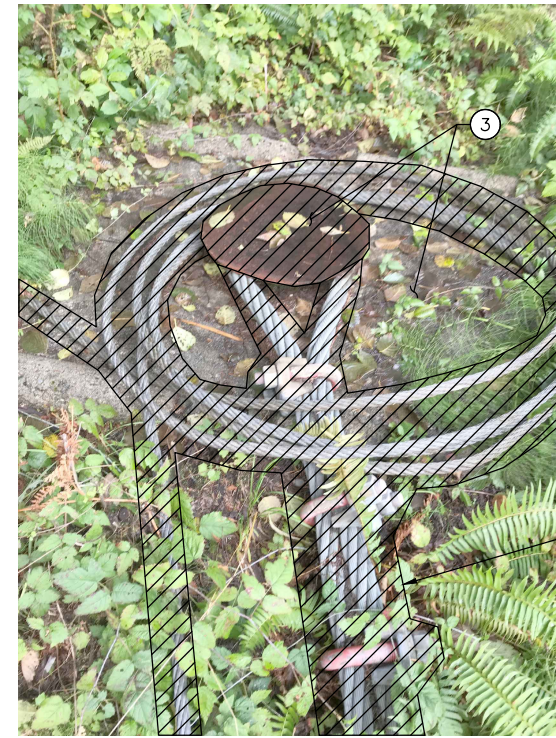
PHOTO – EXISTING RIGHT SHORE ANCHOR
