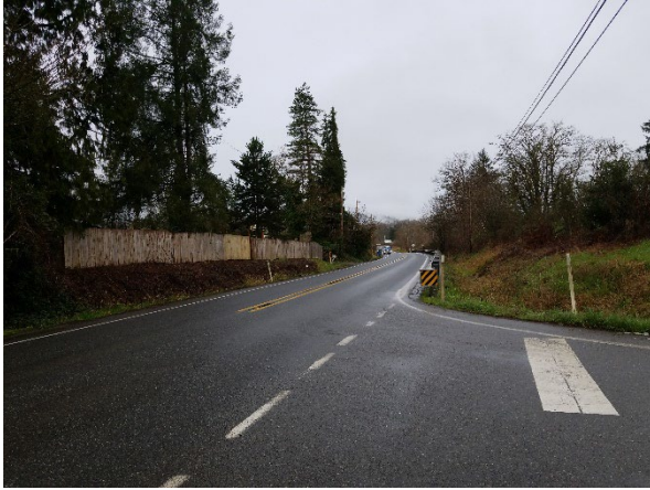
Photo 19. NE 24th Street/SR 203 intersection (HMS 8 proposed location).
