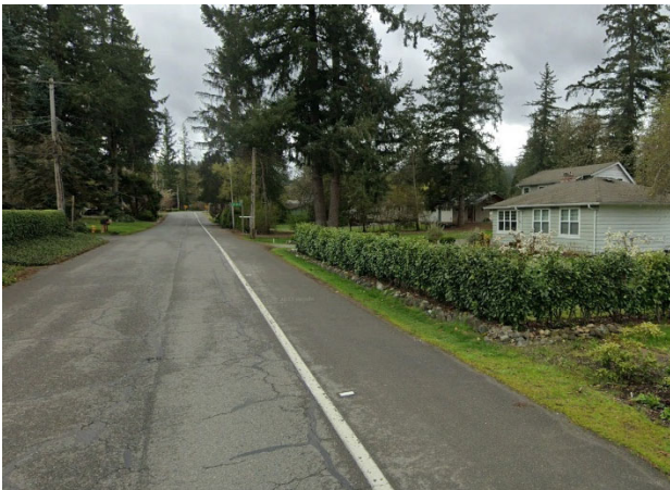
Figure 24. Paved Street without Curb
