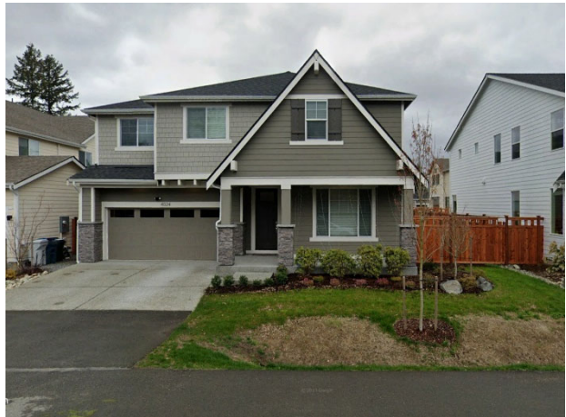
Figure 35. Attached Garage with Driveway Access from the Street
