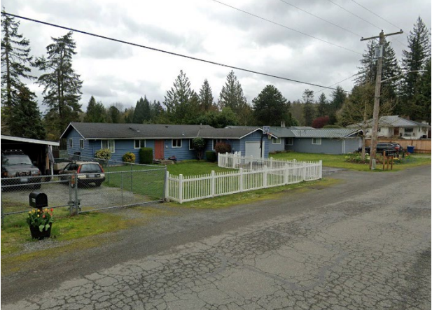
Figure 21. One-Story Ranch Home with Attached Garage
