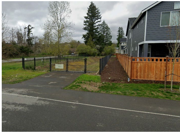
Figure 33. On-site Stormwater Pond
