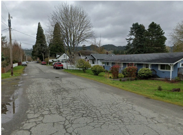
Figure 13. Wide Pave Street without Curbs
