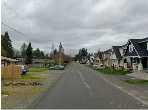
Figure 32. Wide Paved Street without Curbs
