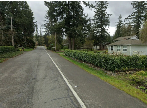
Figure 24. Paved Street without Curb
