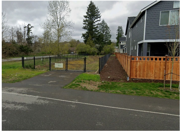
Figure 33. On-site Stormwater Pond
