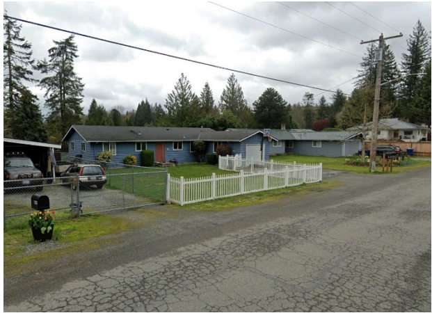
Figure 21. One-Story Ranch Home with Attached Garage
