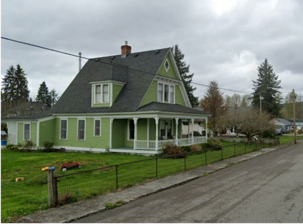
Figure 12. Various Building Styles - Historic Victorian Style Building
