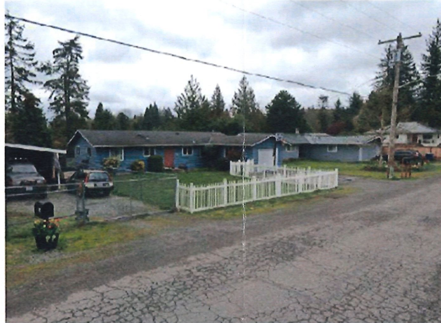
Figure 22. One-Story Ranch Home with Attached Garage
