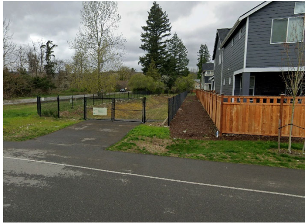
Figure 33. On-site Stormwater Pond
