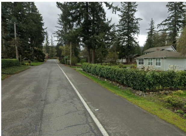
Figure 24. Paved Street without Curb
