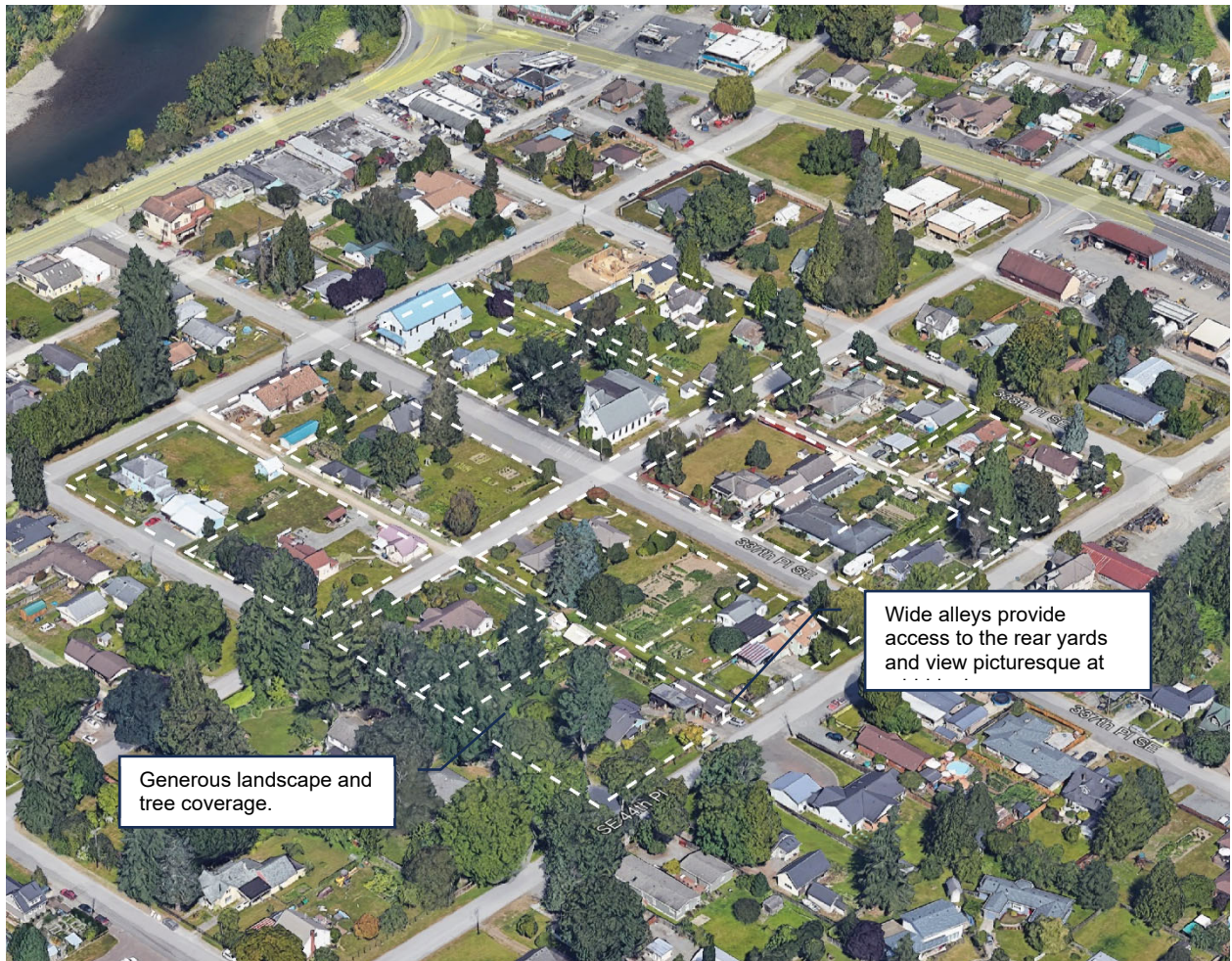
Figure 23. Site 1 Aerial View
