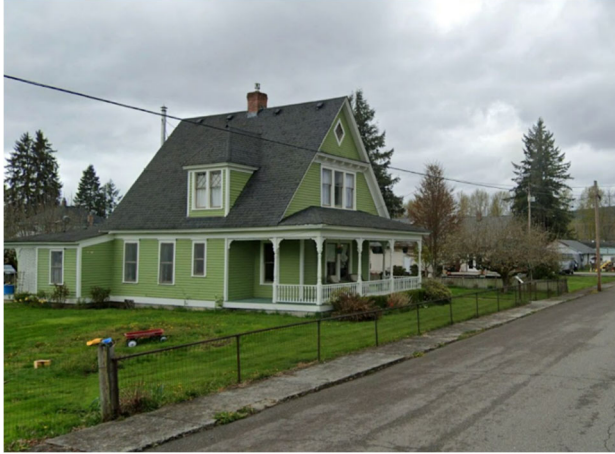
Figure 12. Various Building Styles - Historic Victorian Style Building
