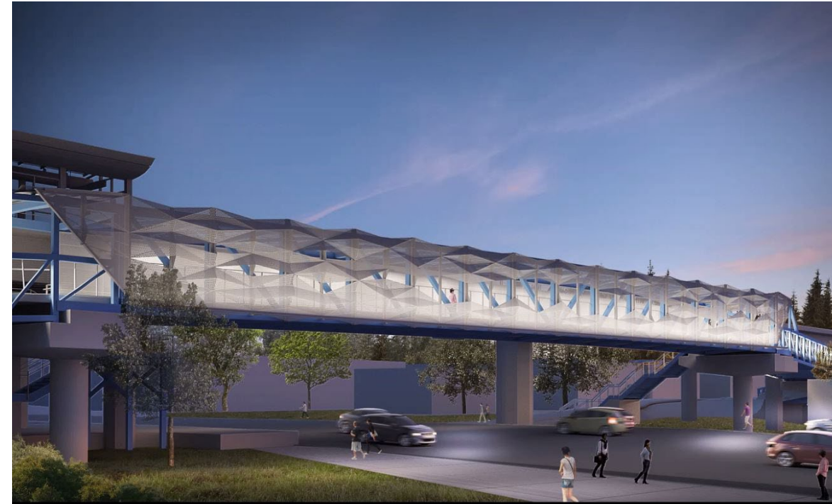
NE 8 th St. crossing
