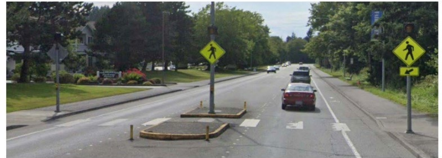
Figure 3-37: Enhanced crossing serving transit stops. This crossing of SR 11 in Bellingham provides a safe crossing opportunity for people accessing the transit stops on either side or other destinations nearby.
