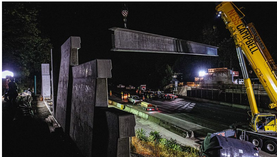
Construction of Eastrail bridge over I-405
