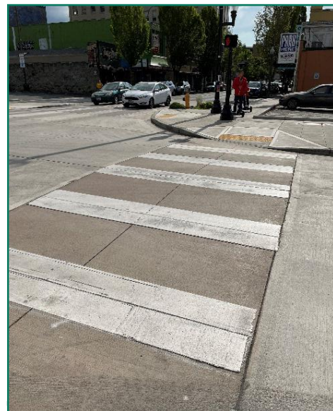
FIGURE 58. ADA CURB RAMP IN OLYMPIA, WA.
