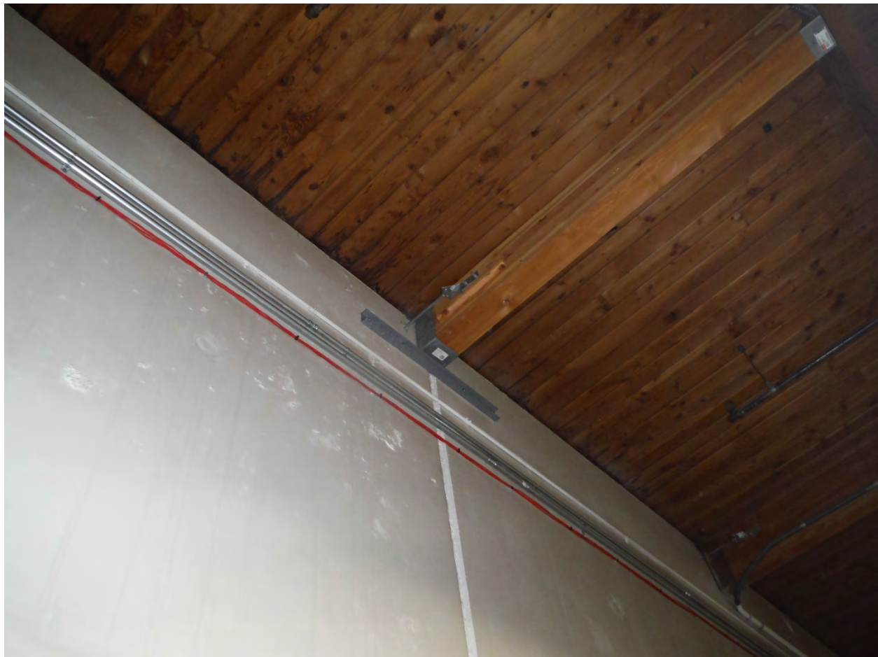
Figure 26. Santler Building – Existing Tilt-Up Wall Retrofits
