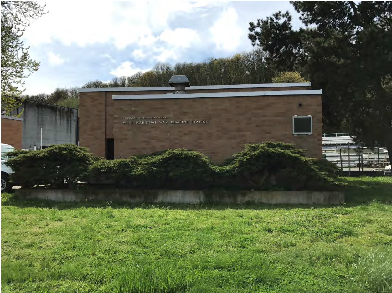
Figure 13. Exterior View of West Marginal Way Pump Station
