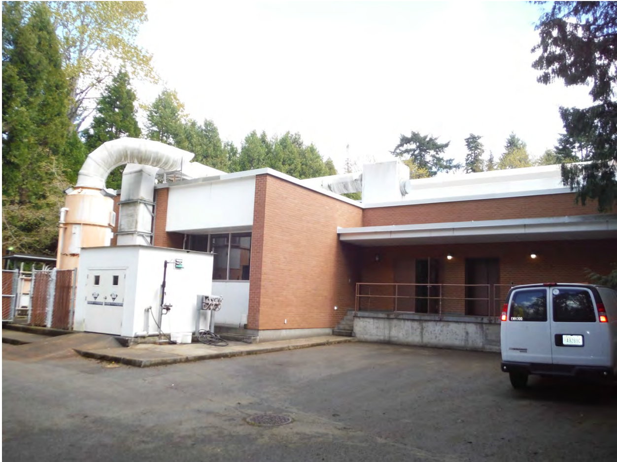
Figure 12. Exterior View of Matthews Park Pump Station
