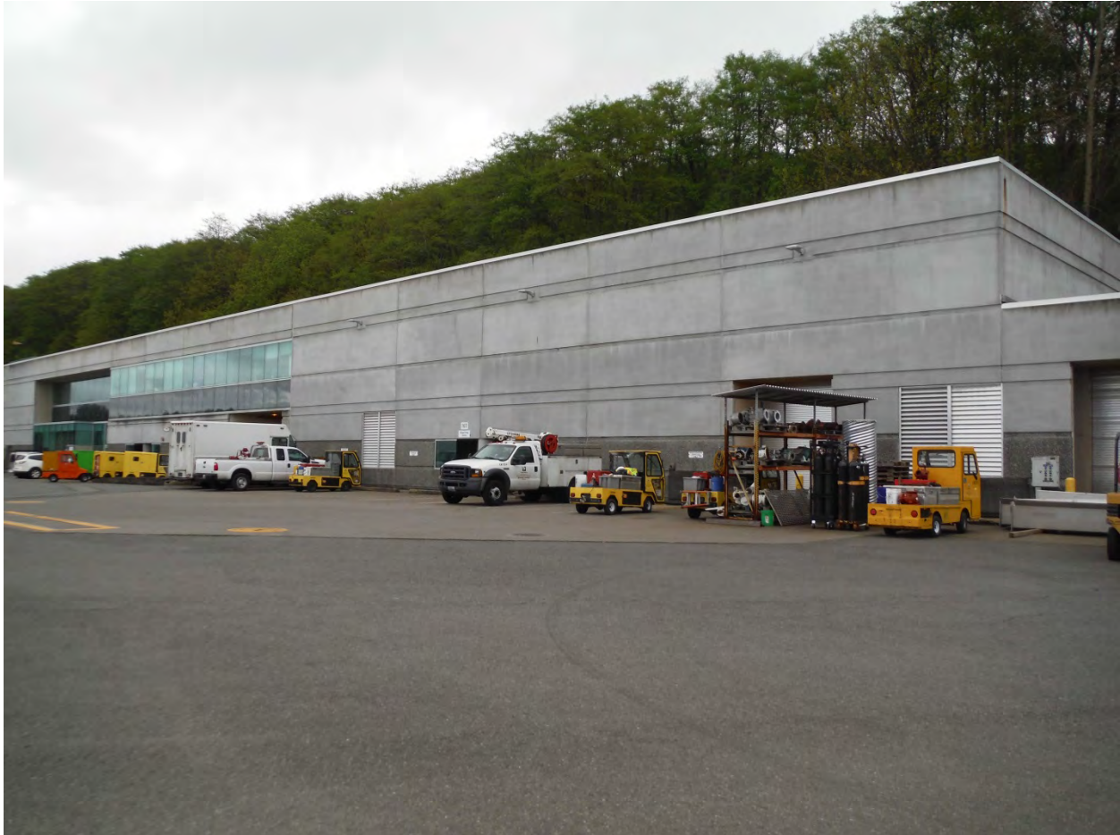
Figure 20. Exterior View of WPTP Maintenance Building (Effluent Pump Station Subgrade Below)
