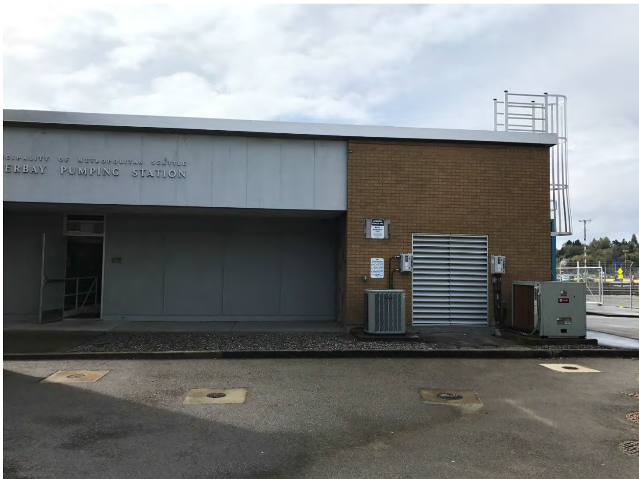
Figure 5. Exterior View of Interbay Pump Station
