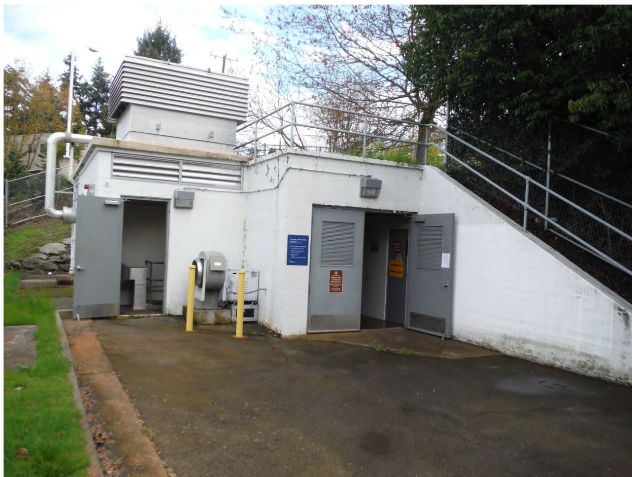
Figure 15. Exterior View of 30 th Ave. Pump Station
