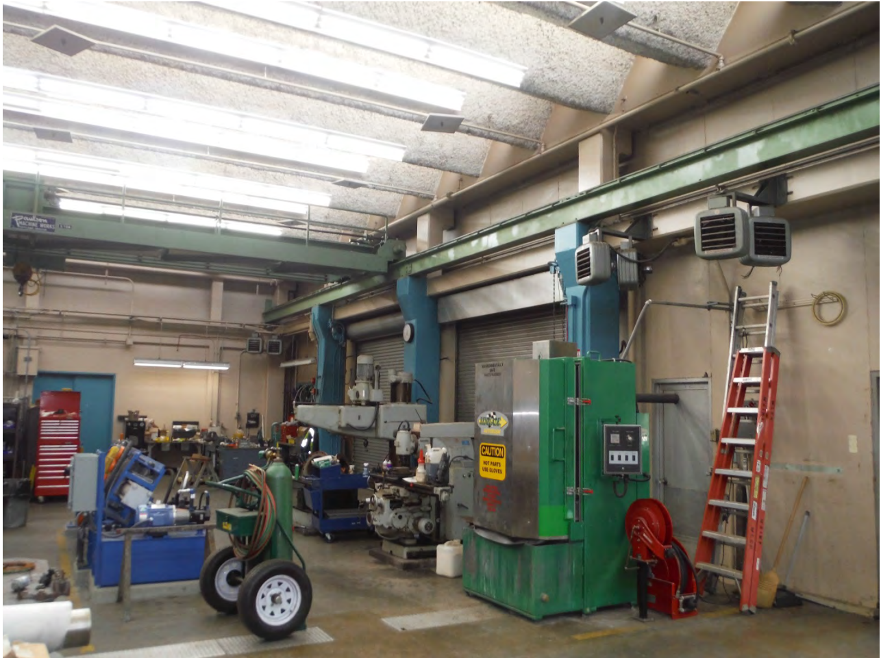
Figure 28. Interior View of STP Maintenance Building, Including Z-Beam Roof
