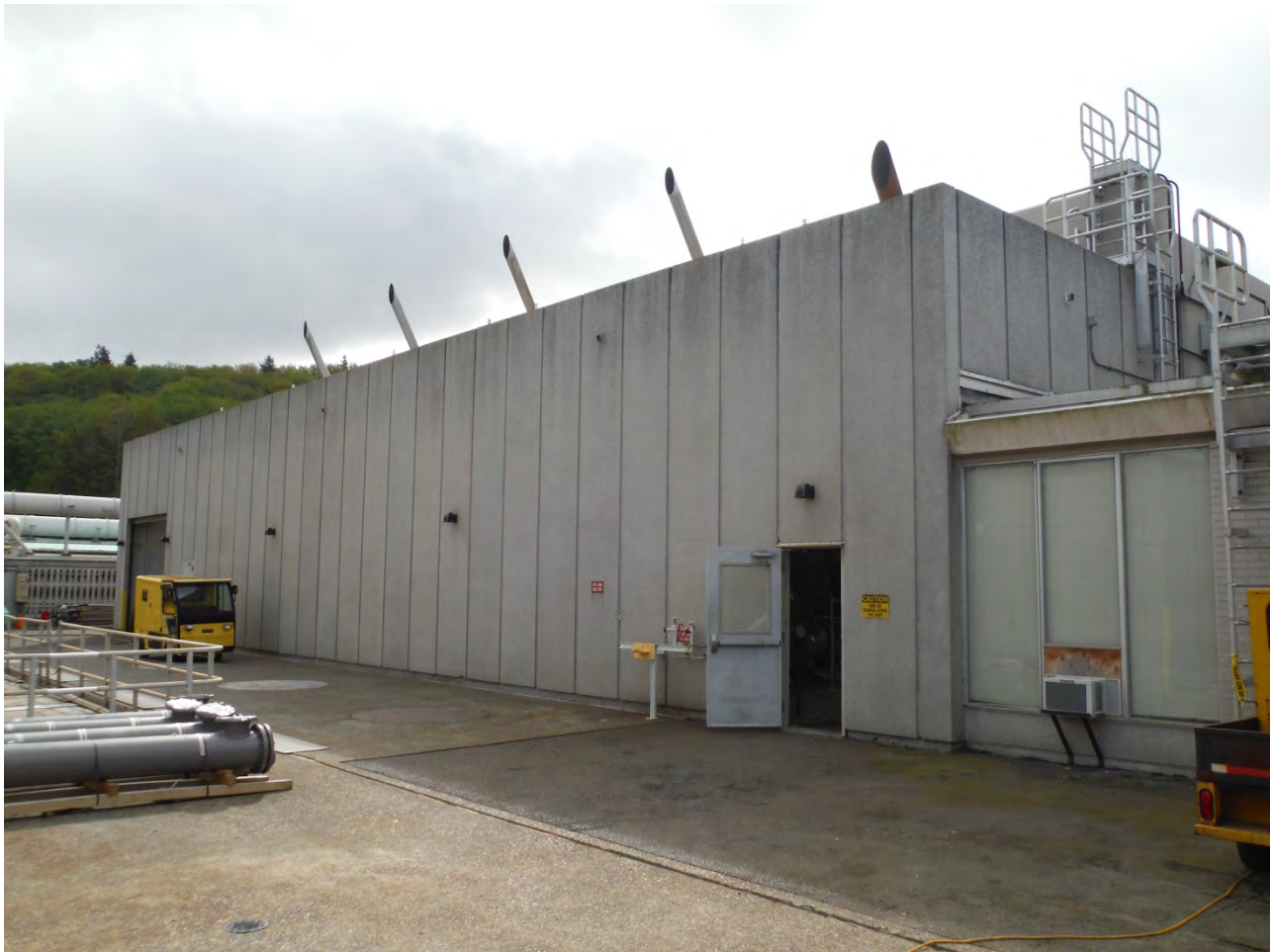
Figure 3. Exterior View of Raw Water Pump Station
