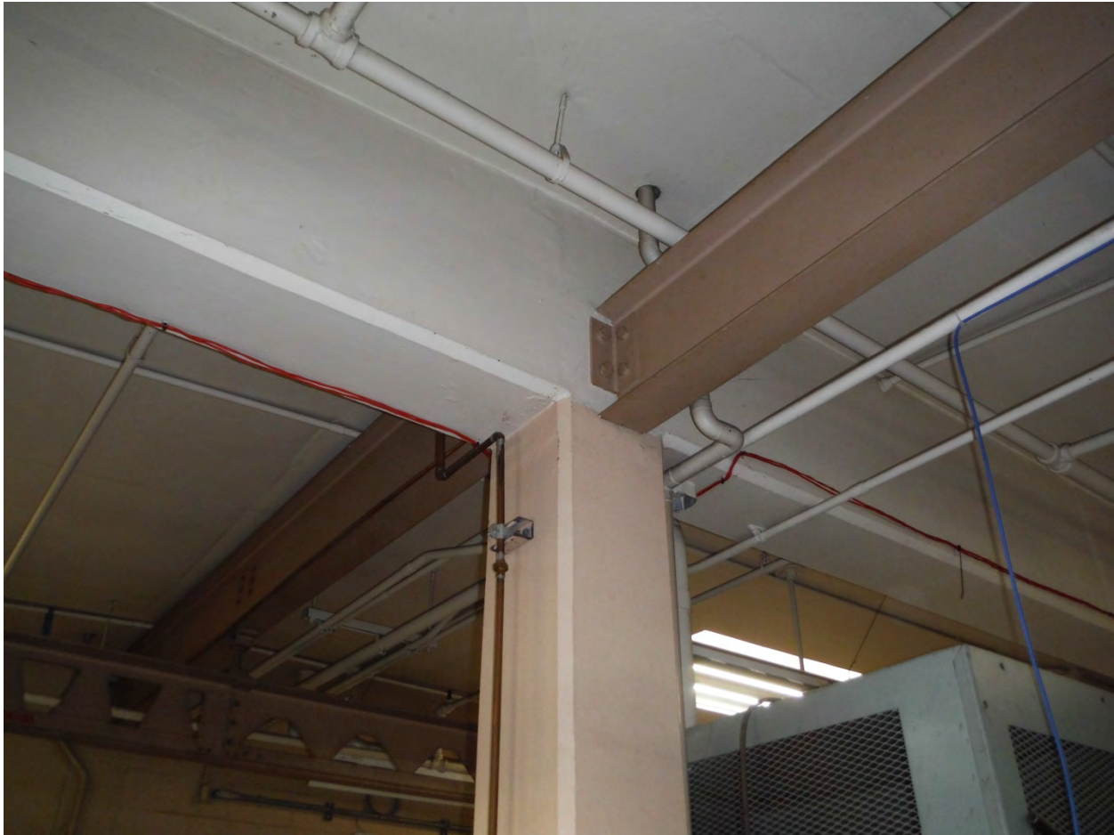
Figure 3. STP Maintenance Building, Weak Column-Strong Beam Framing
