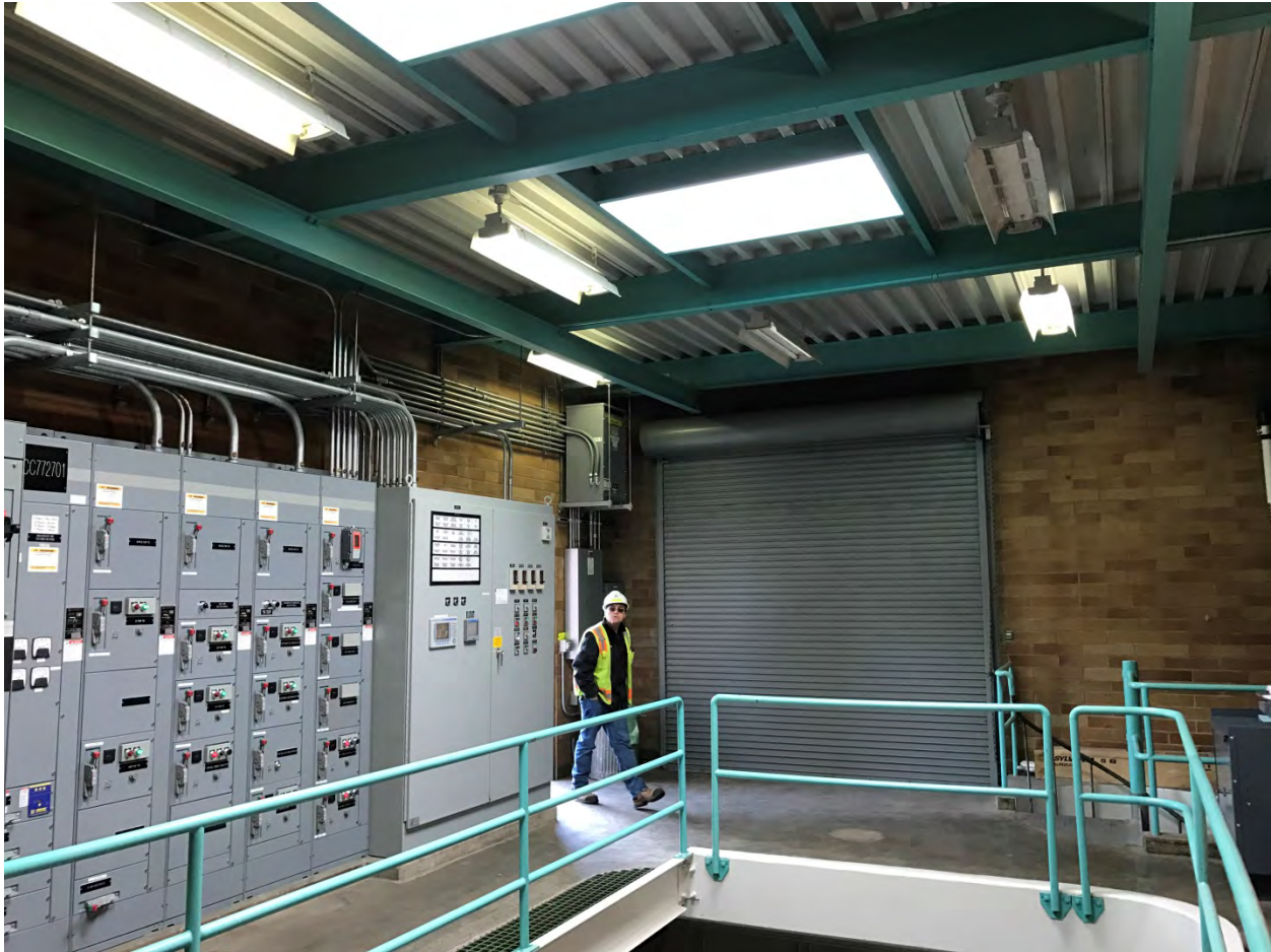
Figure 14. Interior View of West Marginal Way Pump Station, including Diaphragm Openings
