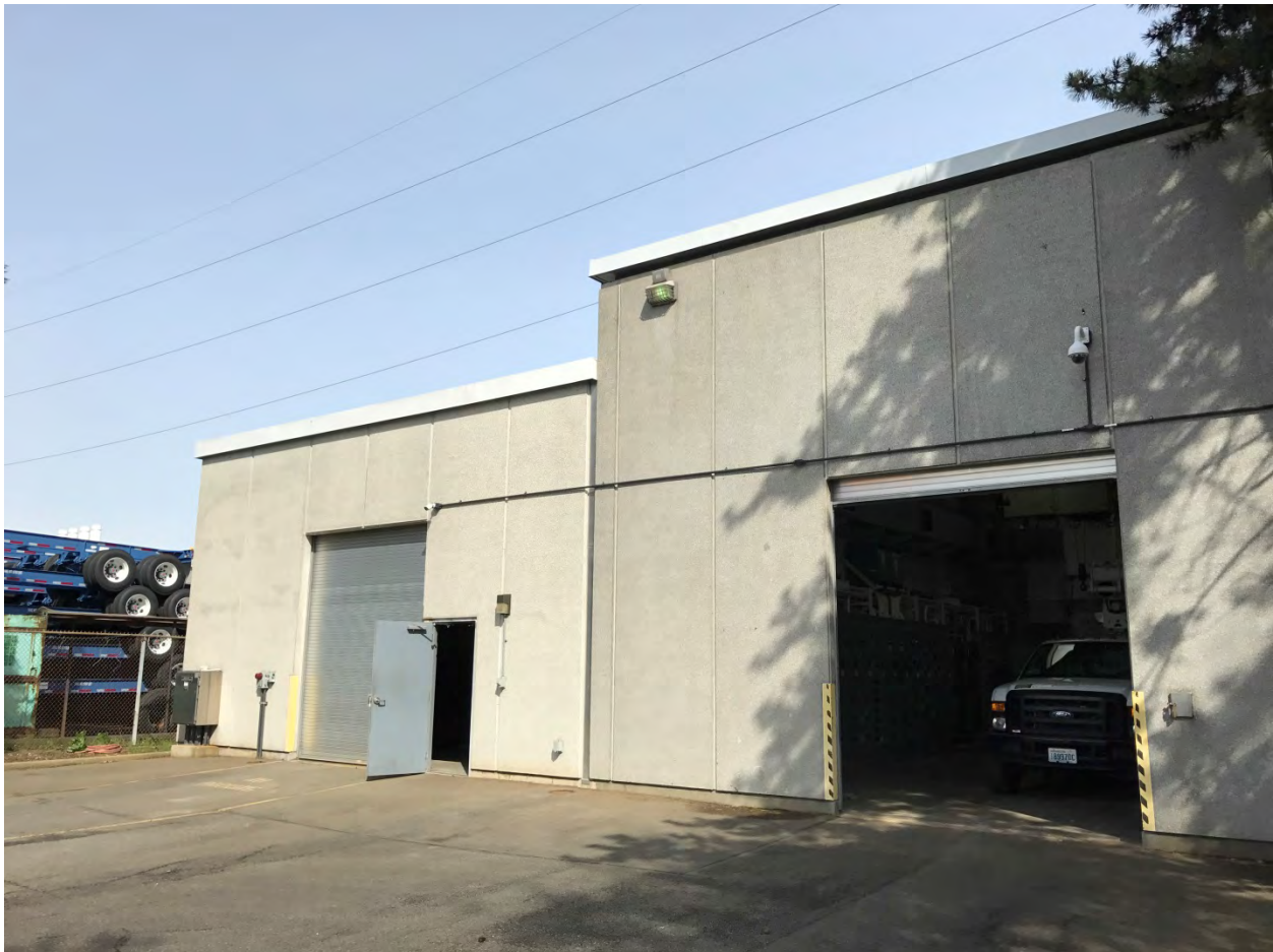
Figure 9. Exterior View of Duwamish Pump Station
