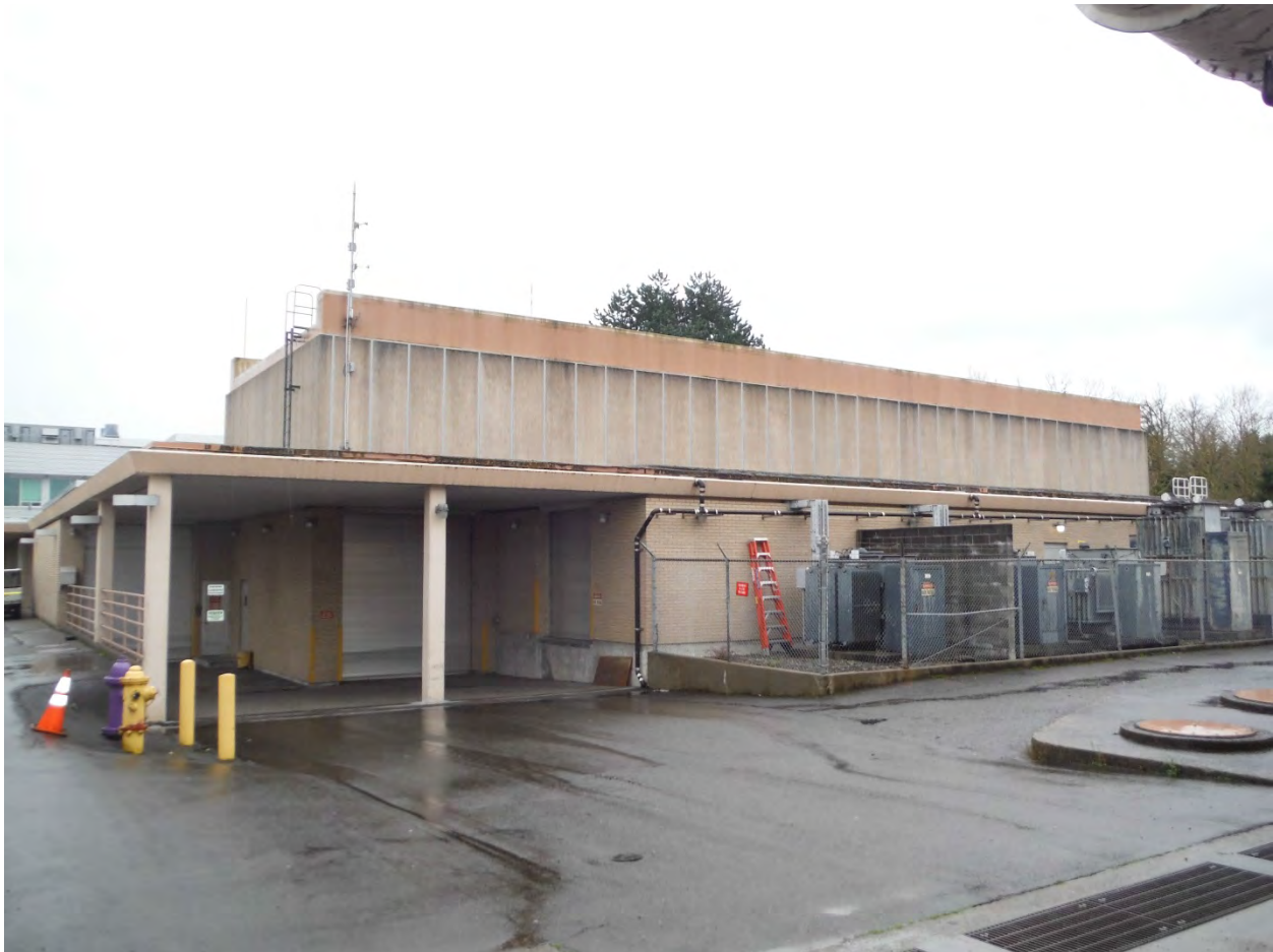
Figure 1. STP Influent Pump Station – Exterior View
