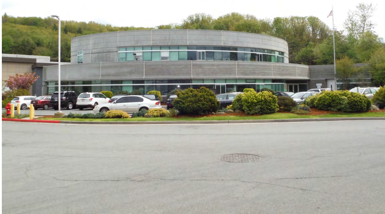
Figure 17. Exterior View of WPTP Admin-Operations Building
