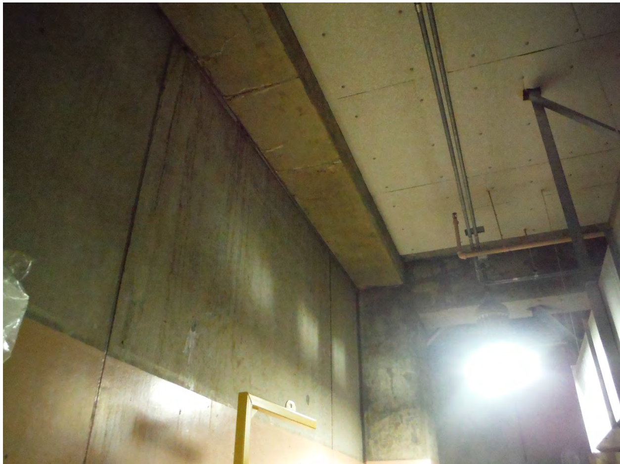
Figure 32. STP Digester Equipment Building, Seismic Joint at Interface with Digesters
