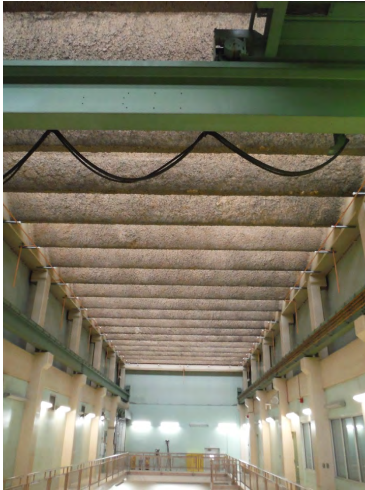
Figure 2. STP Influent Pump Station – Interior View of Z-Beams
