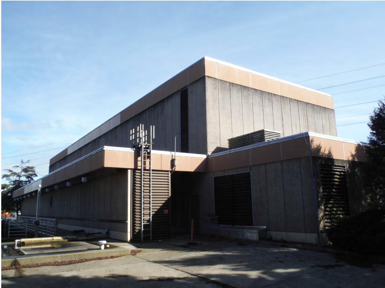
Figure 29. Exterior View of STP Effluent Pump Station
