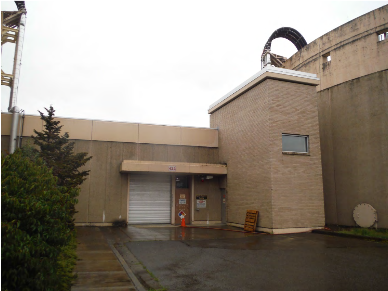
Figure 31. Exterior View of STP Digester Equipment Building (Between four Digesters)
