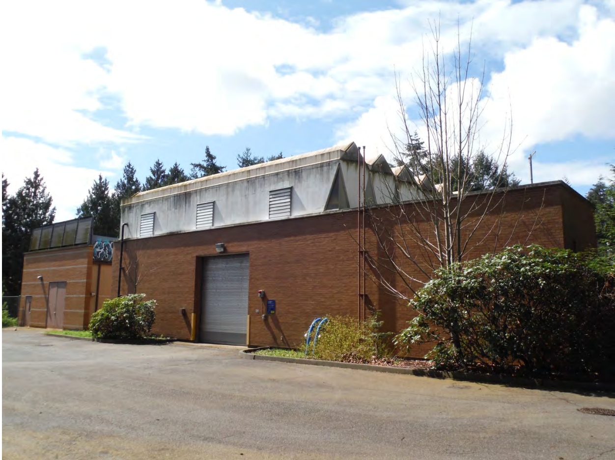
Figure 11. Exterior View of Matthews Park Pump Station
