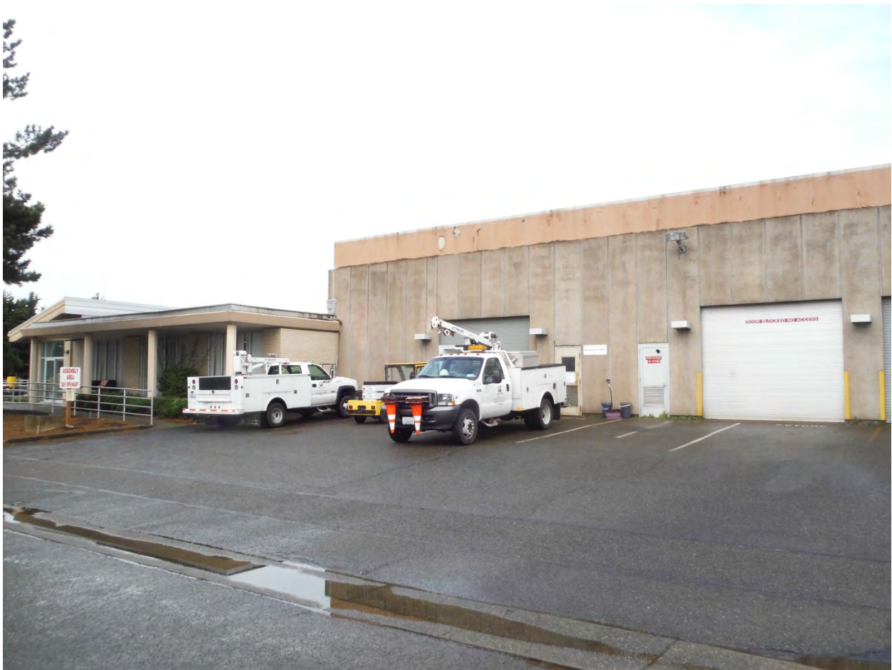
Figure 27. Exterior View of STP Maintenance Building
