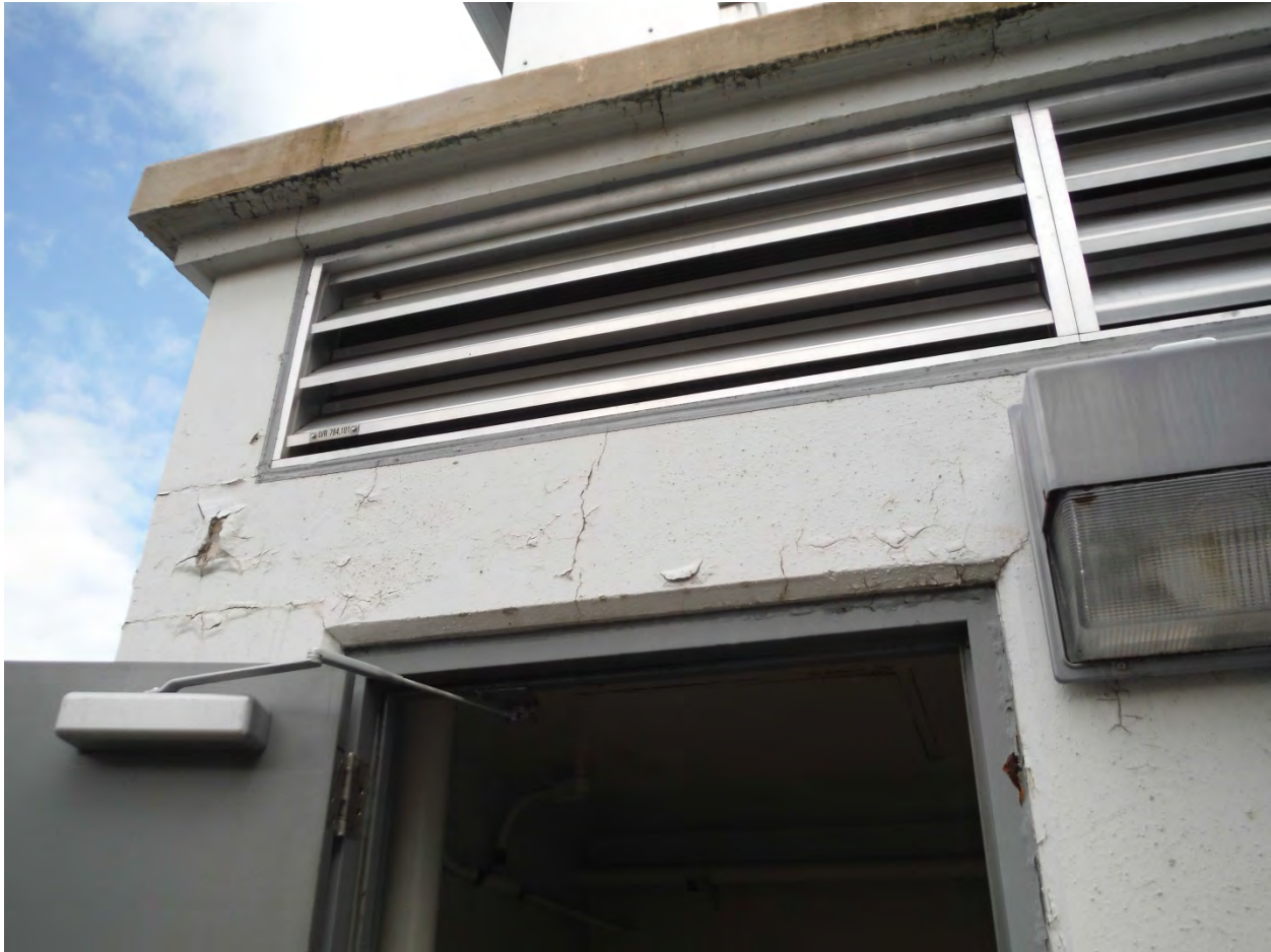
Figure 16. Short Coupling Beam in Poor Condition
