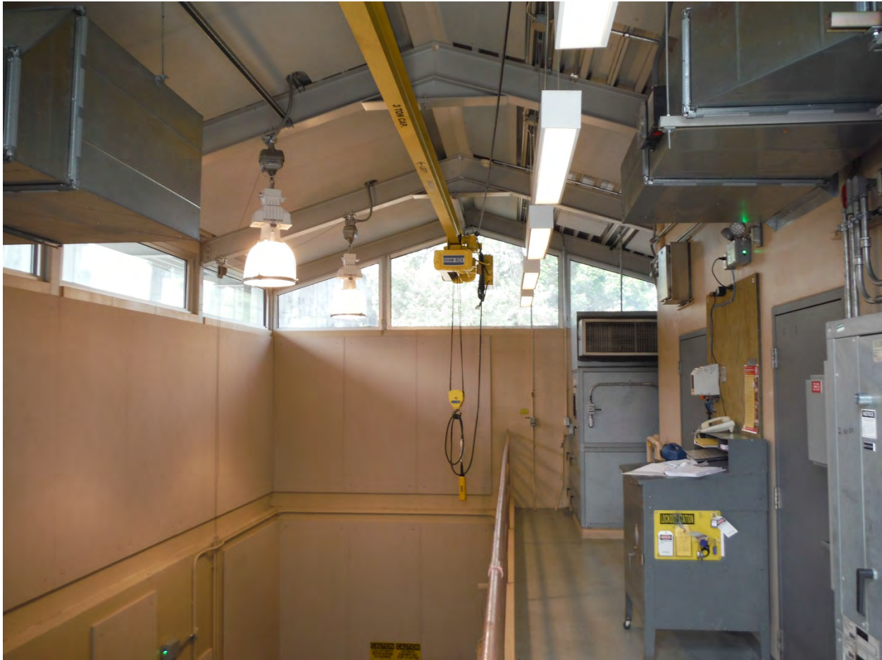
Figure 8. Interior View of Sweylocked Pump Station
