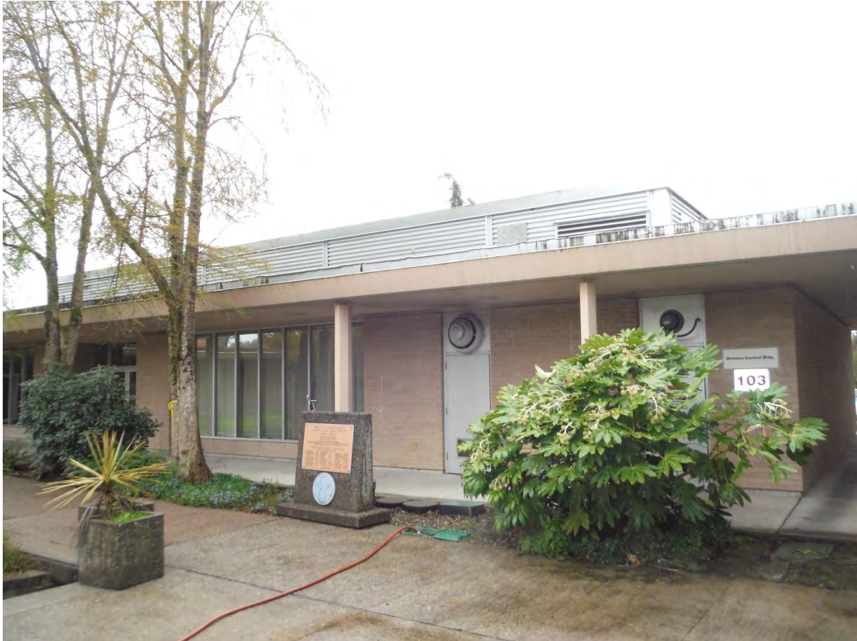
Figure 23. Exterior View of STP Operations Building
