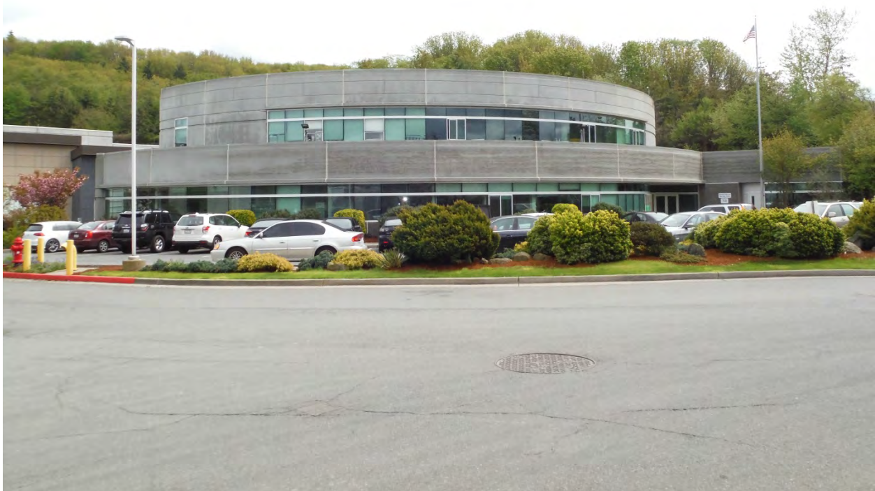
Figure 18. Exterior View of WPTP Admin-Operations Building
