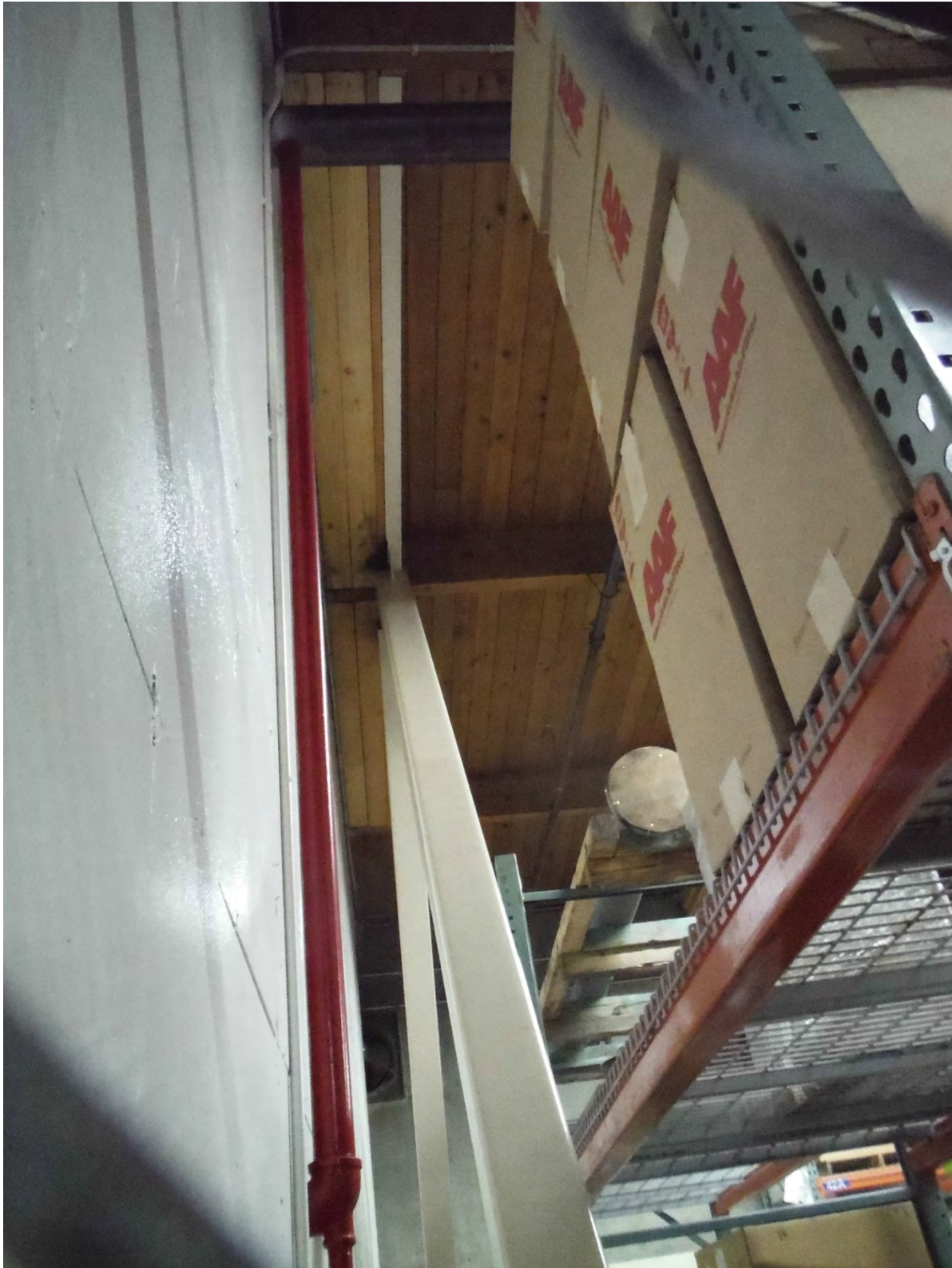
Figure 3. Santler Building – Existing Braced Frame
