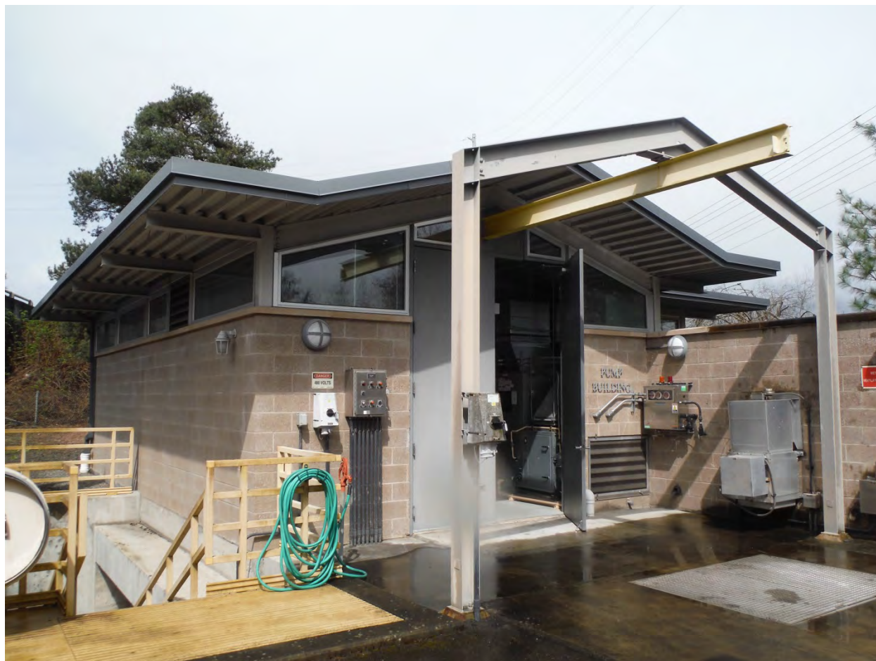
Figure 7. Exterior View of Sweyolocked Pump Station
