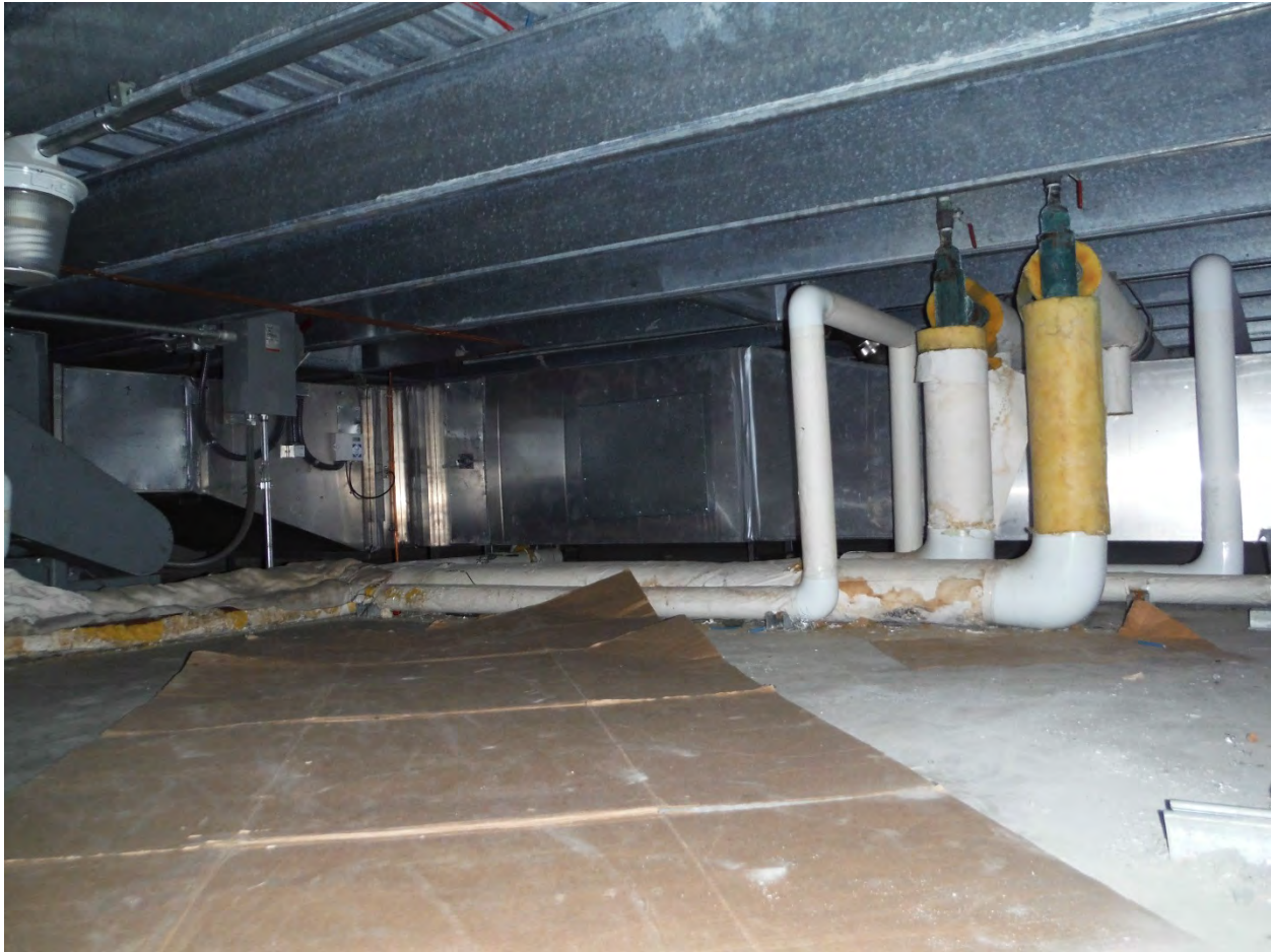
Figure 24. STP Operations Building Mechanical Penthouse Framing
