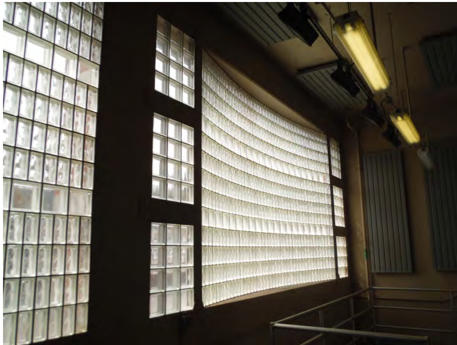
Figure 33. Interurban Pump Station Glass Block Wall Example
