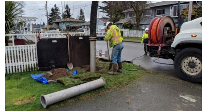
Repair pit for un-inverted liner portion
