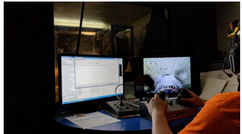
Side sewer reinstatement
