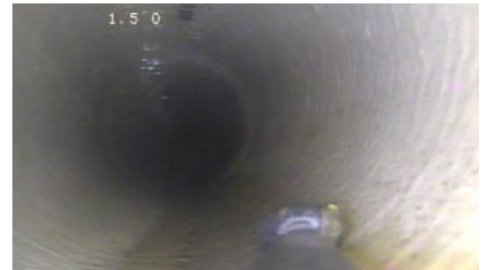
Reinstated upper lateral
