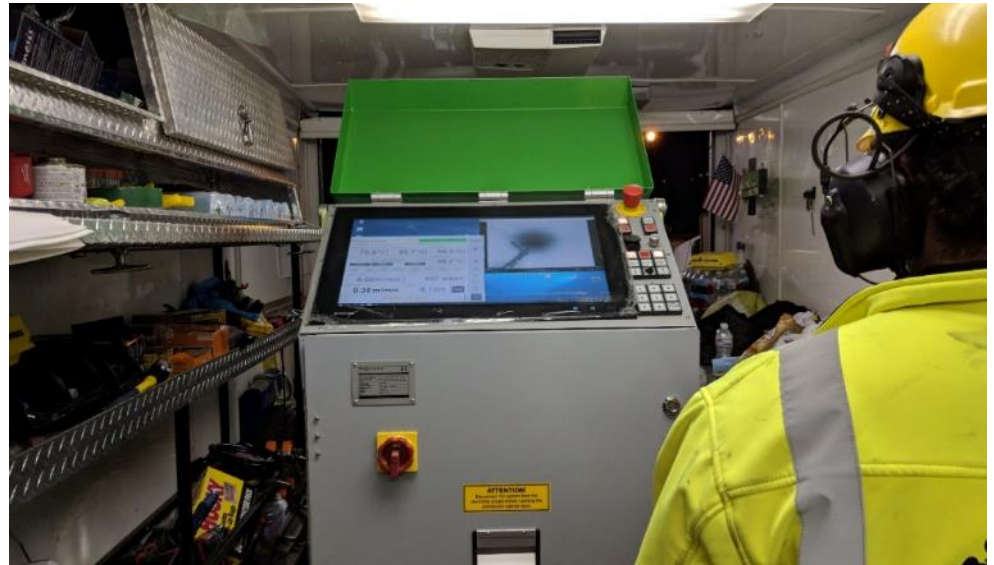
Curing of UV Lining
