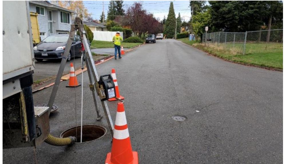
Side sewer location measurement
