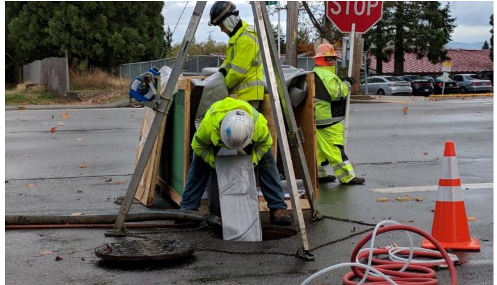
UV liner inserted through manhole
