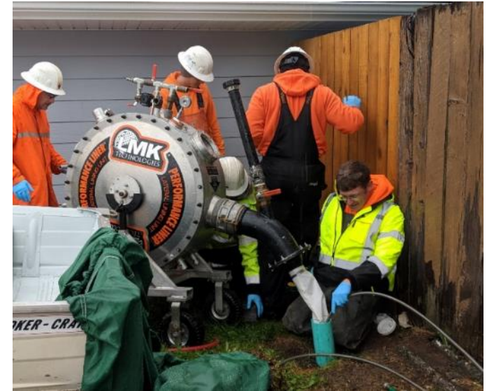
Inserting into cleanout
