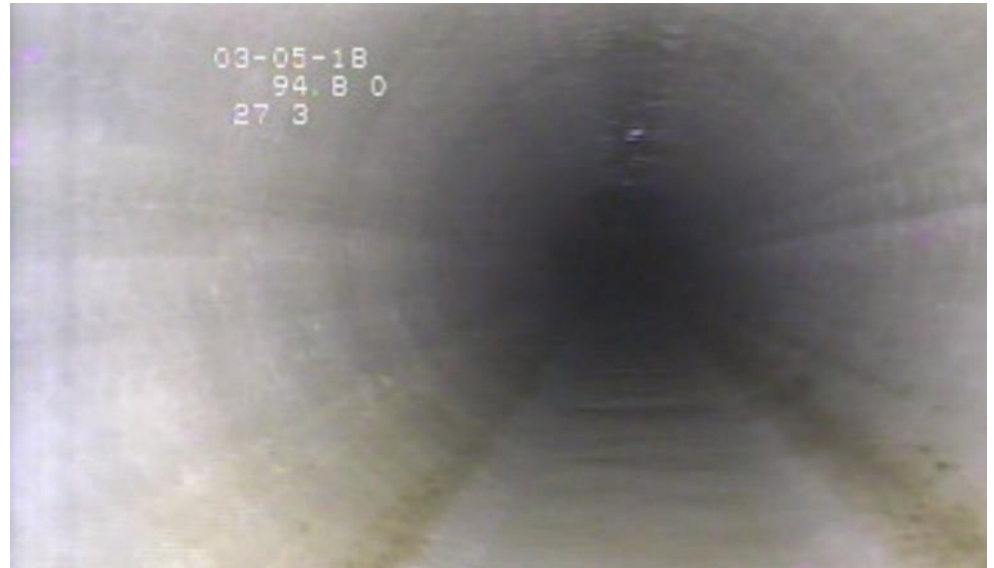
Reinstated Sewer Line
