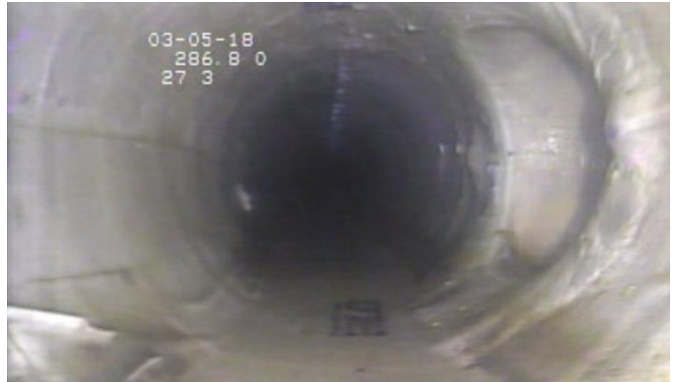
Reinstated lower lateral
