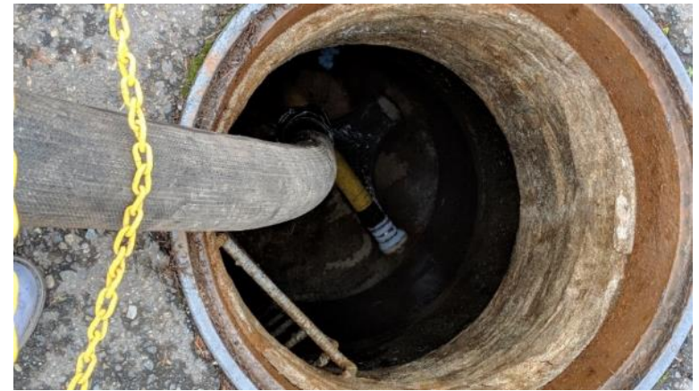
Work near manhole
