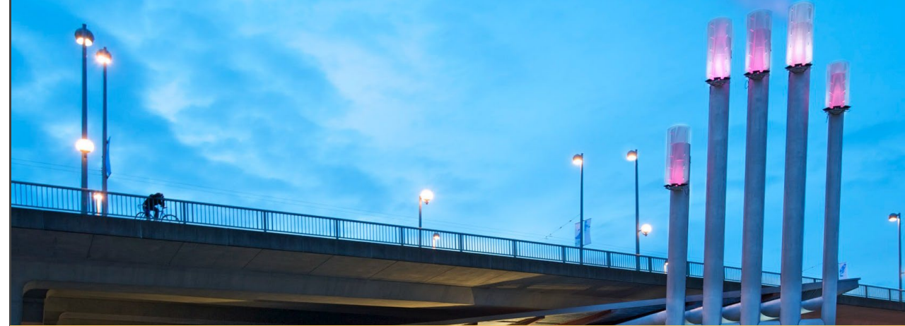
False Creek Neighbourhood Energy Utility, Vancouver BC
