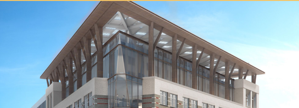
American Geophysical Union HQ, Washington DC
