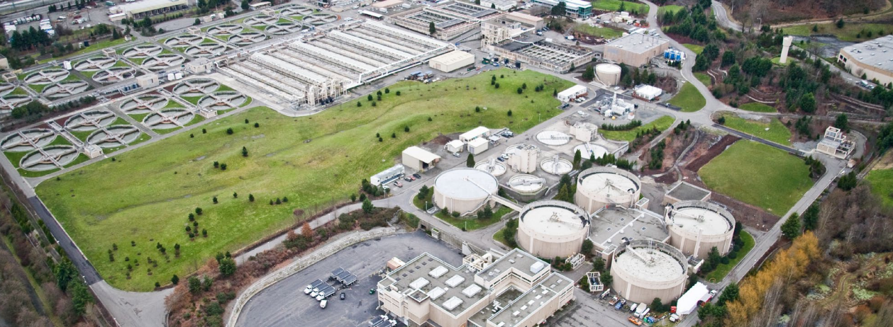
King County South Plant
