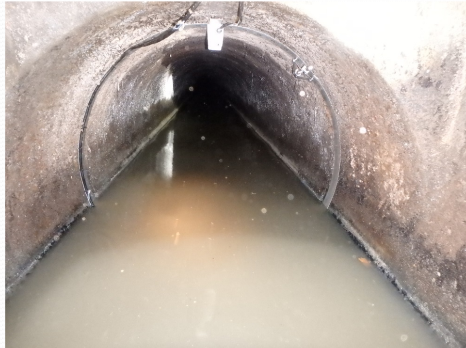
Triton+ Installation with Peak combo and smart depth sensors
