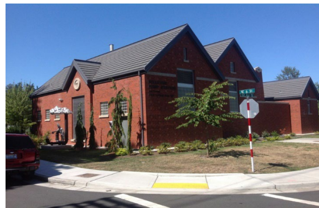
Bellevue Pump Station
