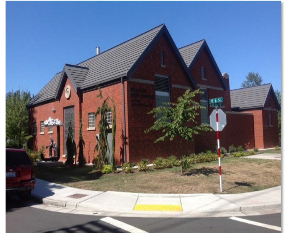
Bellevue Pump Station
