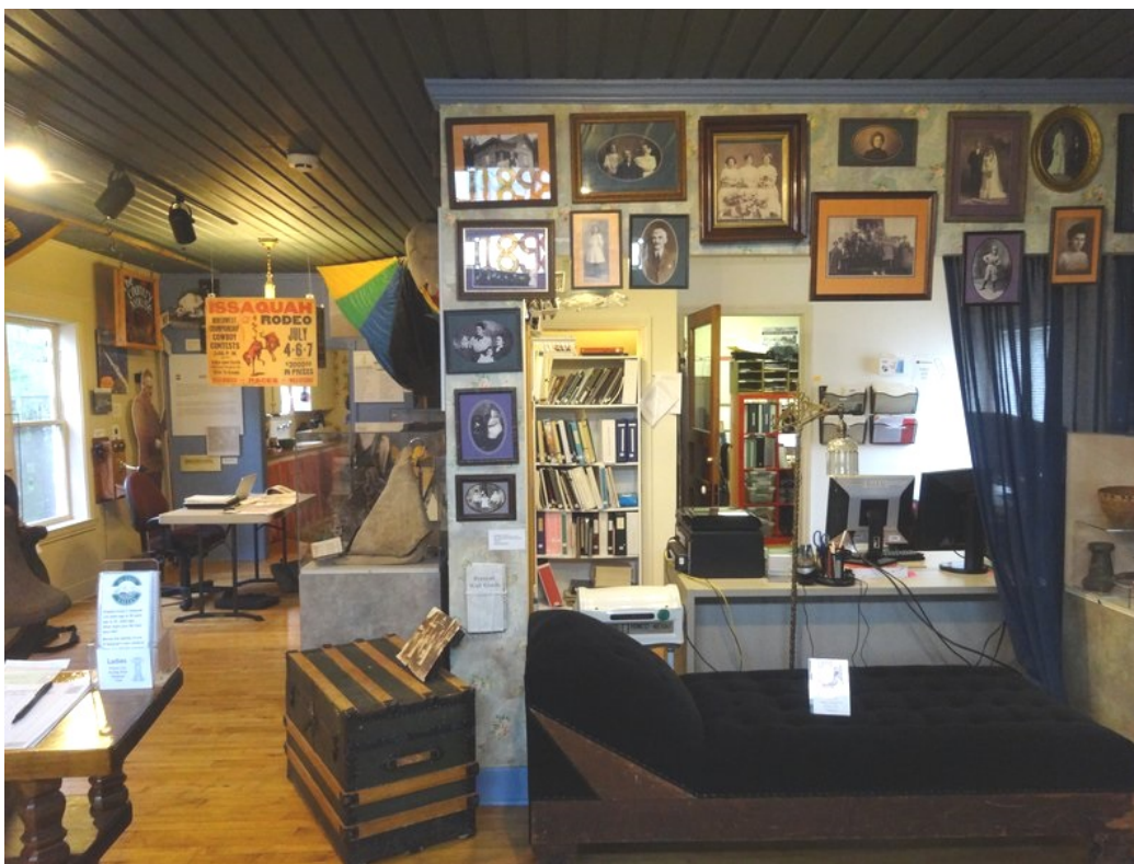
Figure C10. Town Hall interior, research room, showing beaded tongue-in-groove sheathing on west wall. Camera facing southwest.
