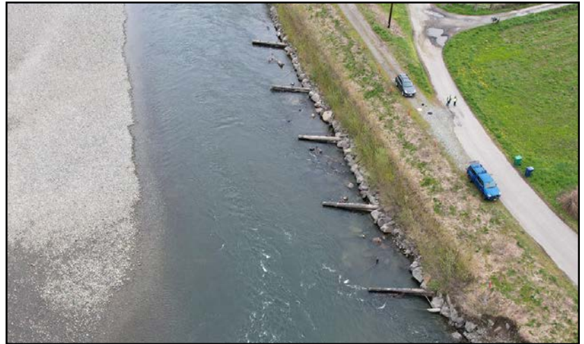
Example of a river revetment.
