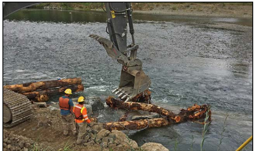
2019 revetment repair on the Snoqualmie River downstream from Stossel Bridge.
