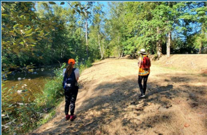
Levee inspection in progress
