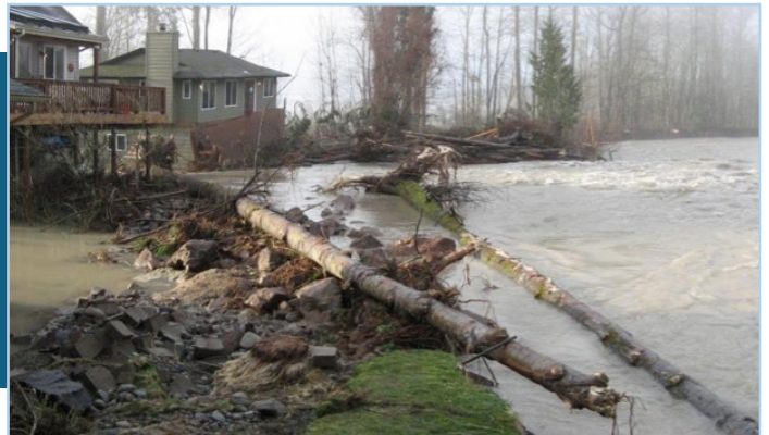
Tolt River levee breach, January 2009
