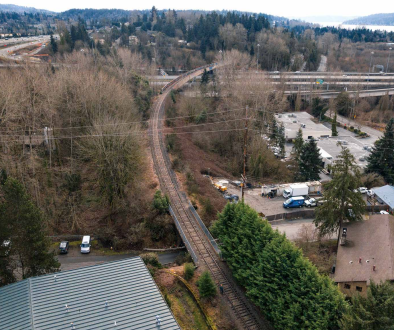
FIGURE 15. RAIL AT 32ND TRESTLE LOOKING SOUTH
