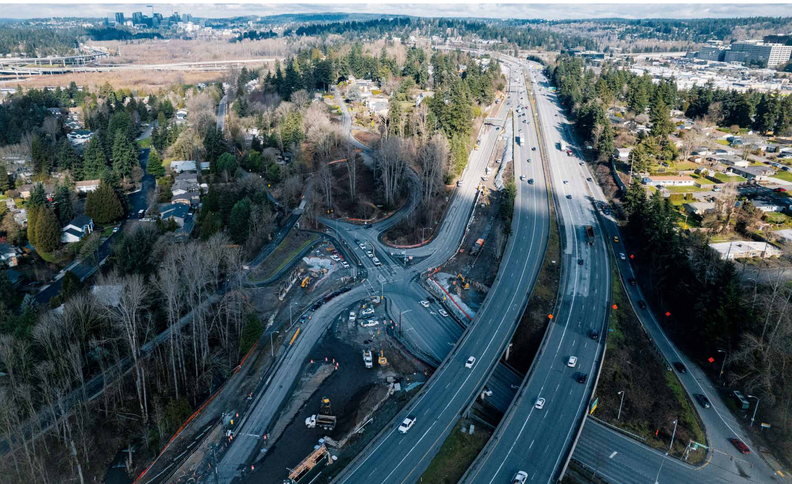
FIGURE 14. EXISTING CONDITIONS – COAL CREEK PARKWAY LOOKING NORTH
