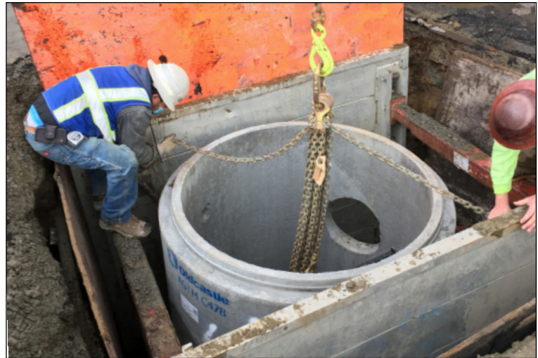
Relocating utilities prior to trail construction.
