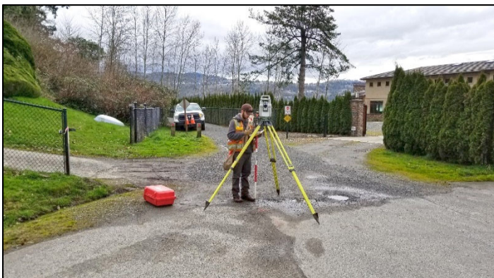
Conducting final surveyors updates on the ELST South Sammamish B segment.
