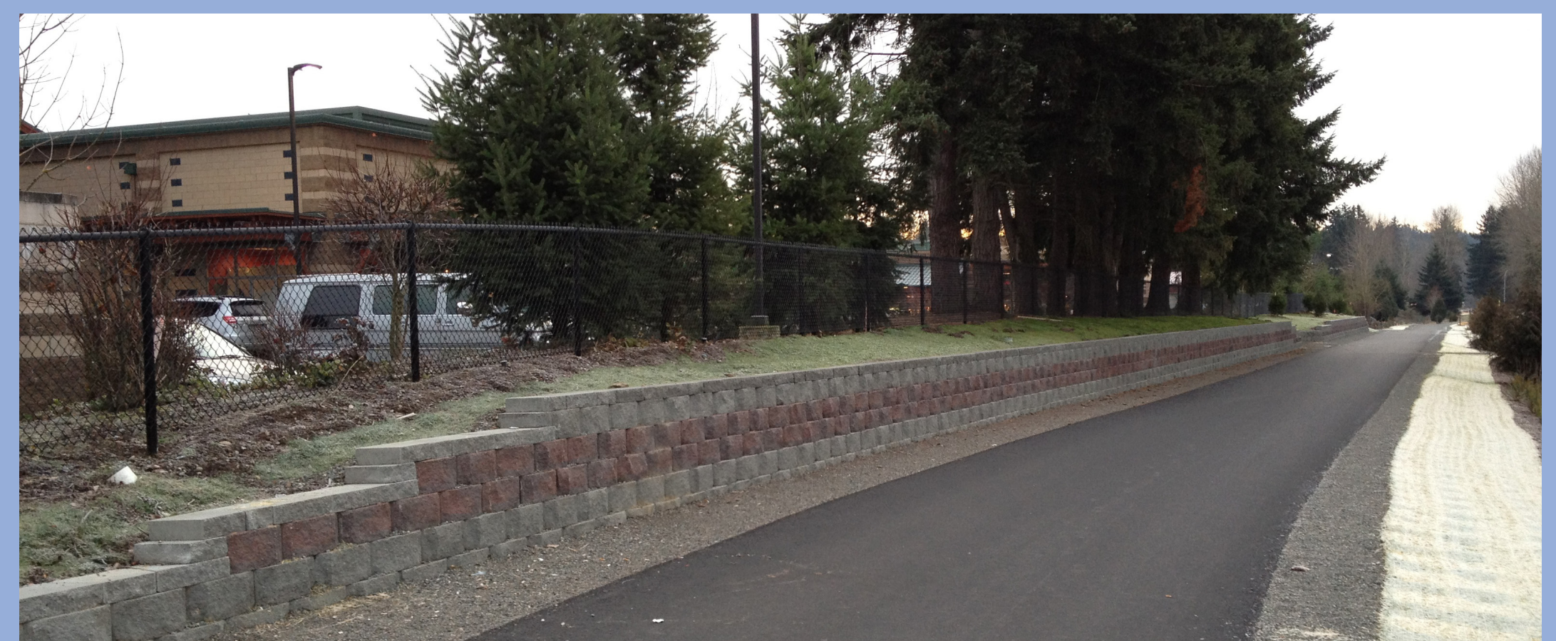
Retaining walls are installed to minimize impacts to environmentally sensitive areas, or to reduce the size of the project footprint, minimizing impacts to adjacent properties.
