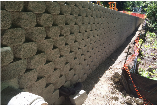
Completed Structural Earth Wall
