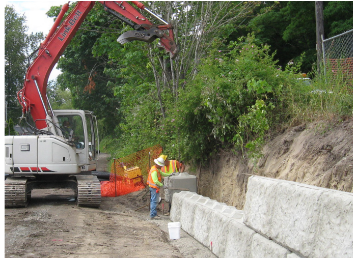
Construction of a gravity block wall
