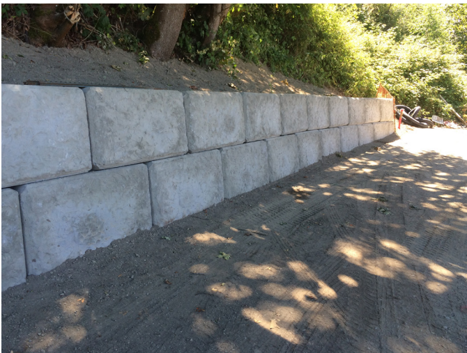
Completed Gravity Block Wall
