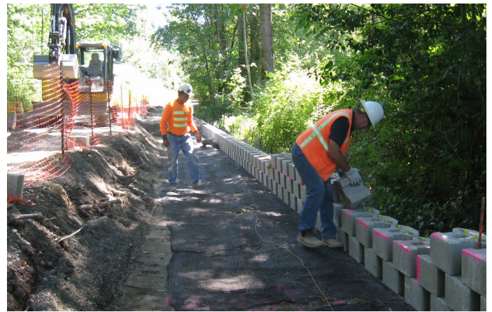
Construction of a Structural Earth Wall
