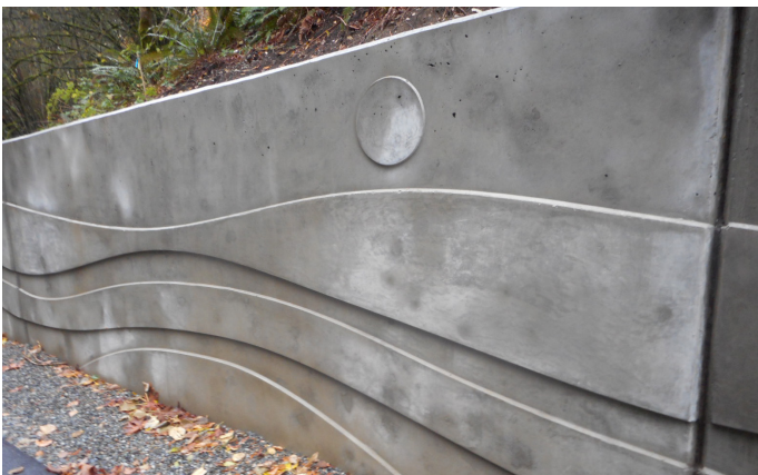
Completed soldier pile wall
