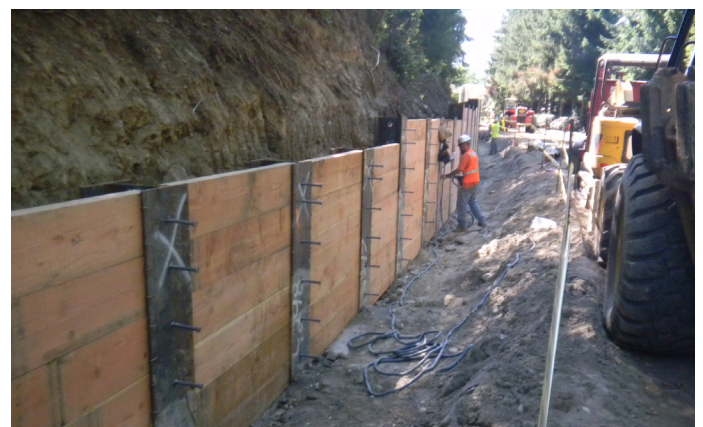
Construction of a soldier pile wall
