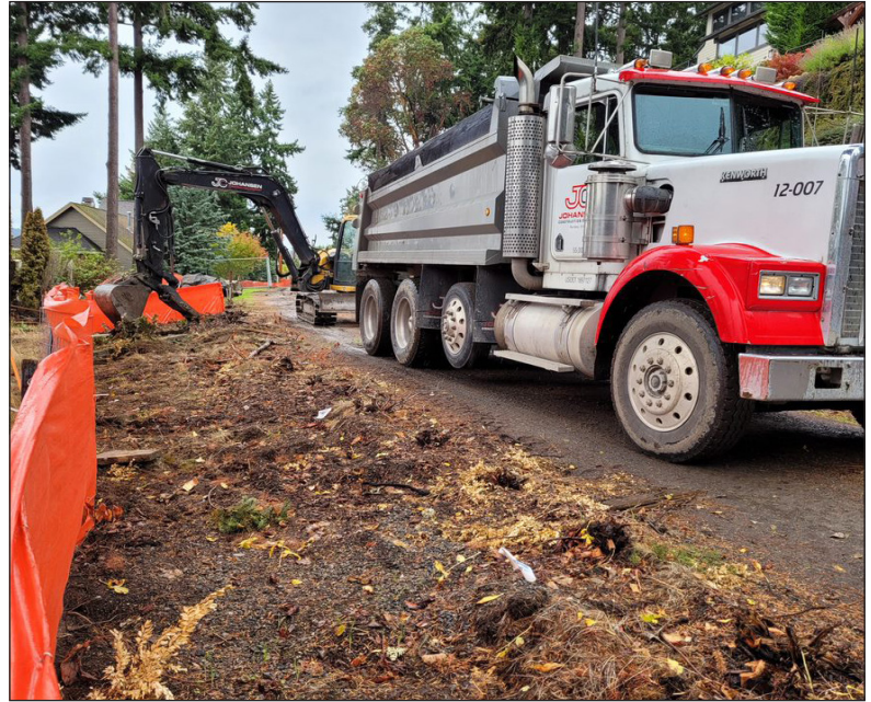
Crews begin grubbing, removing stumps and roots of previously cleared vegetation.
