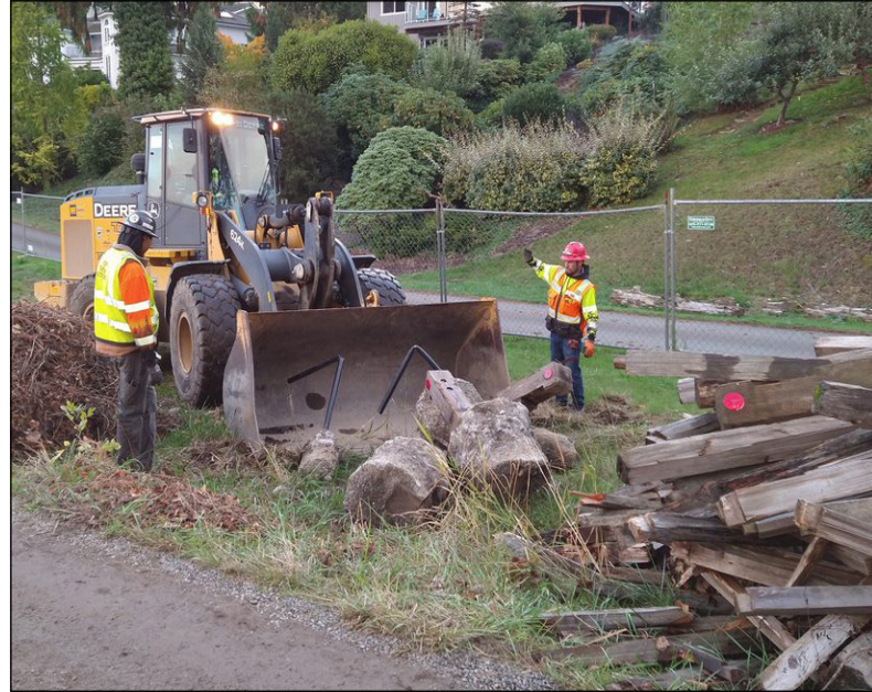
A team loads cleared guardrails and posts during clearing and grubbing activities.
