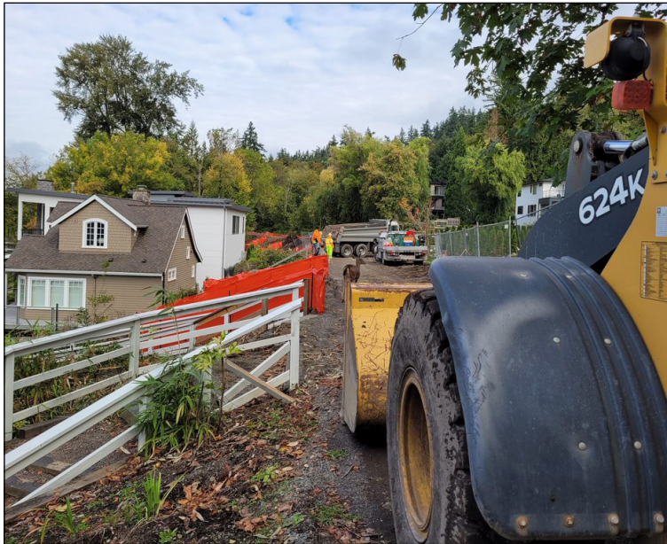
Trailside view of a bucket loader supporting grubbing operations. Most construction vehicles require the full trail width.
