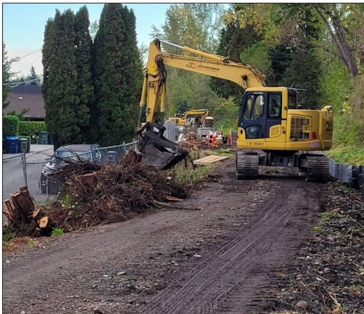
An excavator pulls stumps out of ground to prepare the site for a future retaining wall.
