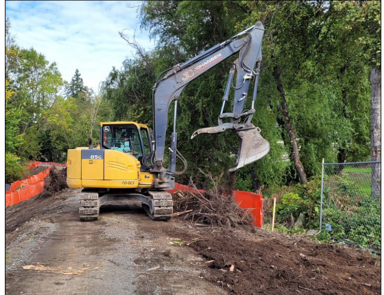
An excavator preparing to load grubbed roots into an awaiting dump truck.
