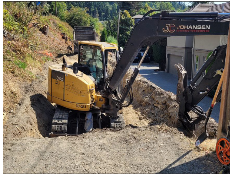
Excavating for the first of many retaining walls to support the new, wider trail.
