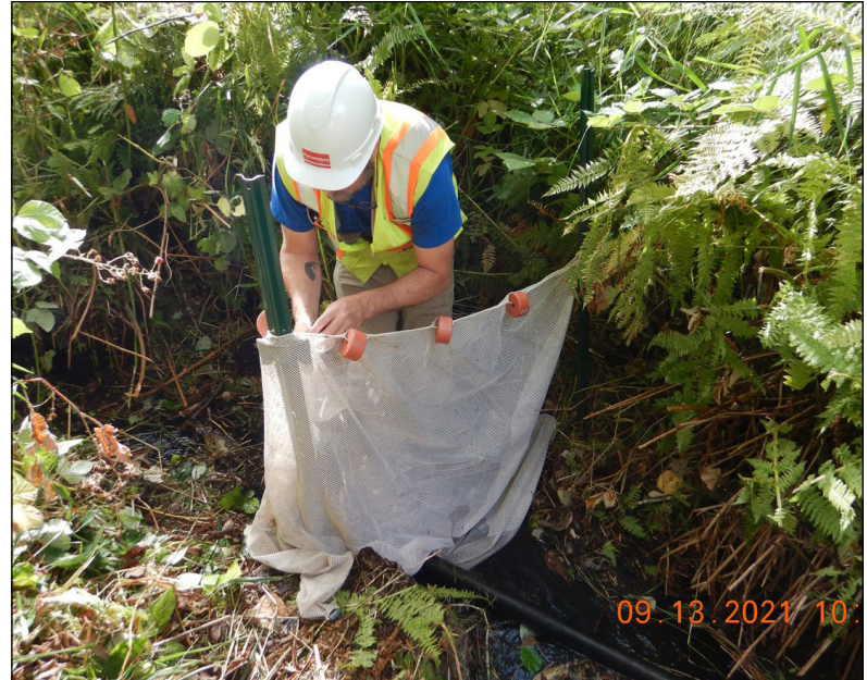
Installing a fish exclusion net upstream of upcoming drainage work. Another net will be installed downstream of the project.
