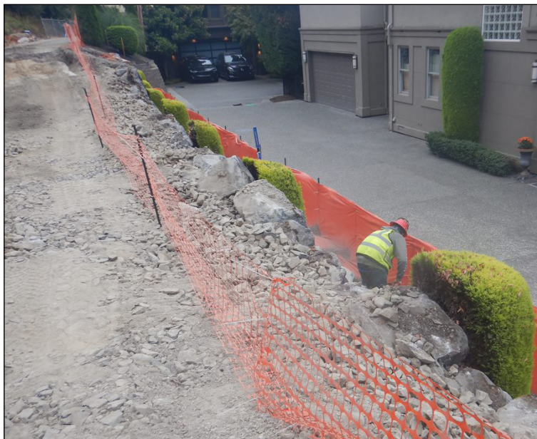
Installing high visibility silt fence below an existing rock wall that will be removed and replaced to widen the trail.
