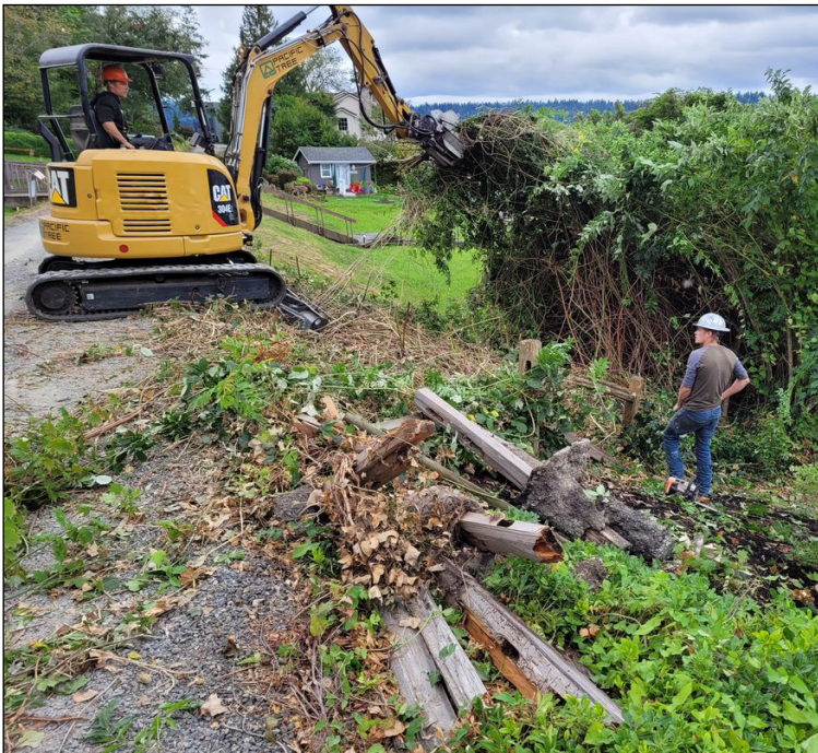
Trailside vegetation and wood fencing is carefully cleared by hand and excavator ahead of earthwork.
