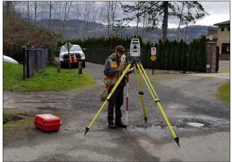
Survey to mark construction limits
