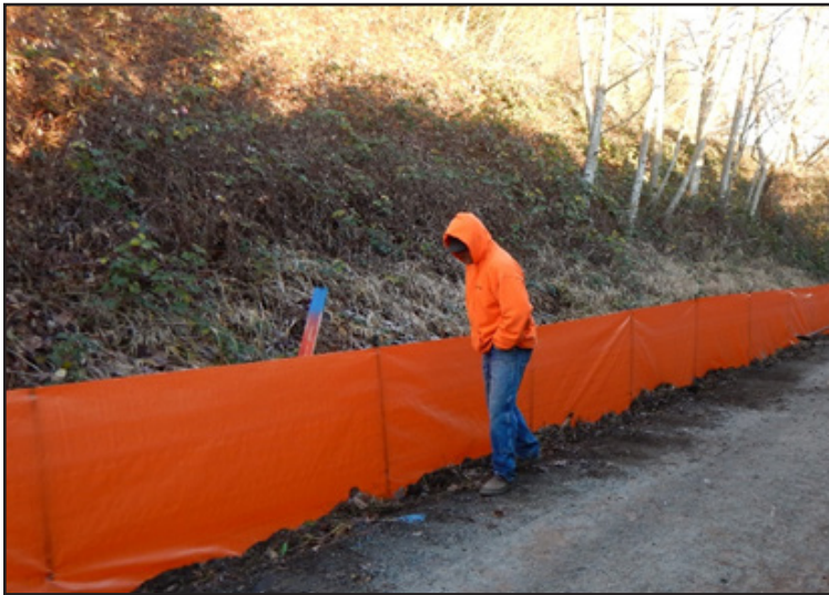
Example of erosion control fencing
