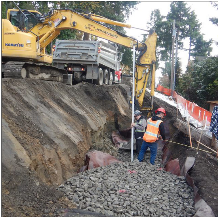
Crews check the depth and width of the trench's rock base as an excavator continues to work behind them.
