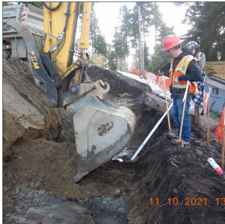
A team member guides the excavator operator as they carefully excavate for a retaining wall, working on a slope and around buried utilities.
