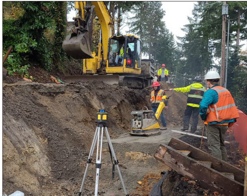
Crews compact gravel as it is installed as the base for a retaining wall's footing, while a geologist monitors the soils being excavated.
