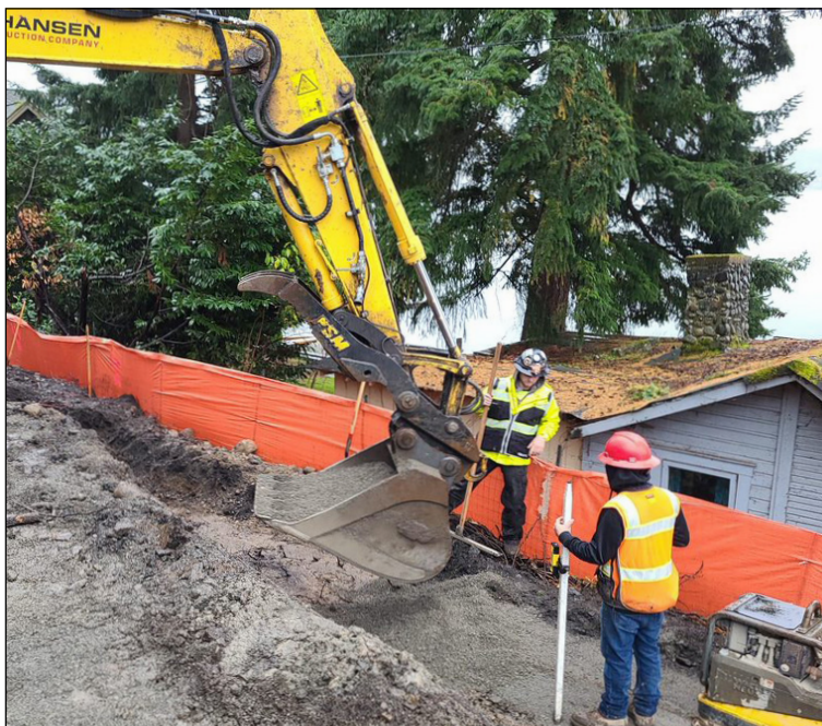
An excavator digs the trench for the retaining wall's footing while a worker checks the excavation depth.
