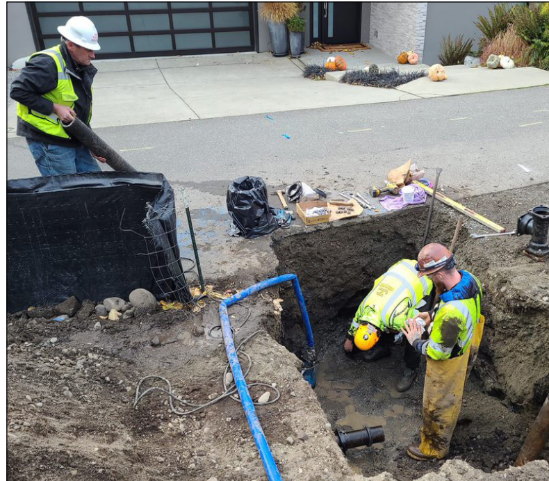
A team relocates a section of water main to make room for a retaining wall's footing.
