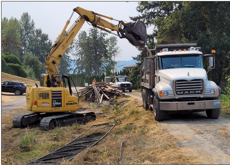
Loading concrete and other debris for removal.
