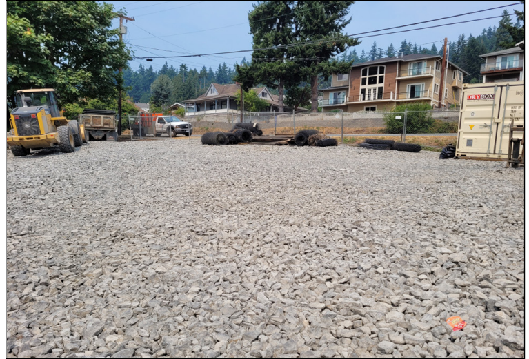
Quarry spall rock installed over geotextile at the SE 33rd Street staging area stabilizes the soil to prevent runoff.
