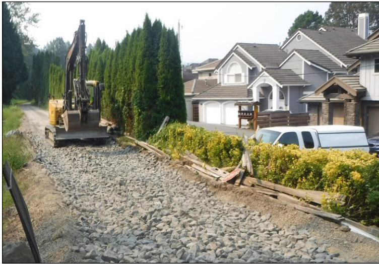
A stabilized construction vehicle entrance was added near the north end of the project.
