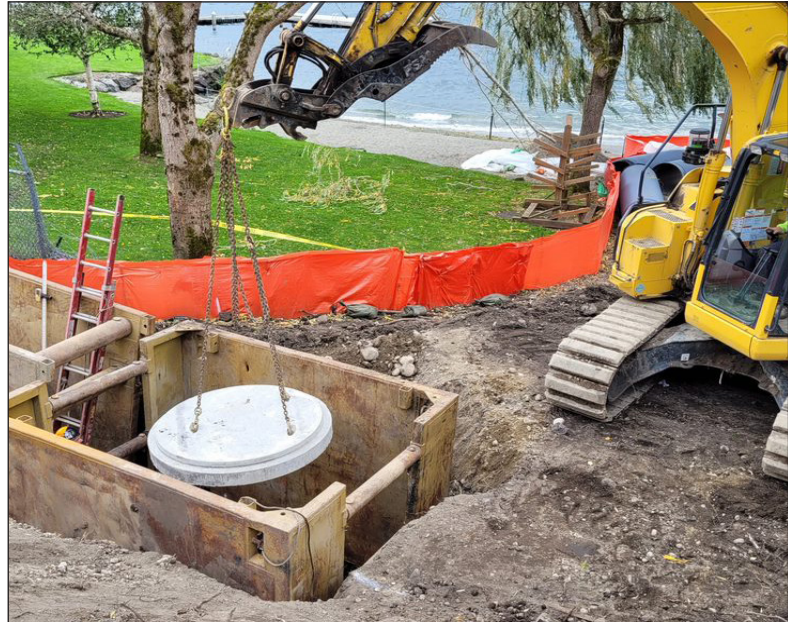
Lowering the base of a drainage structure into place. Metal shoring boxes protect the trench from sloughing during construction.
