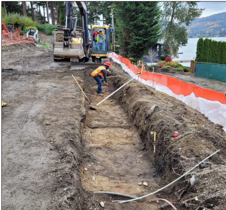
An excavator digs the trench for a retaining wall's footing.
