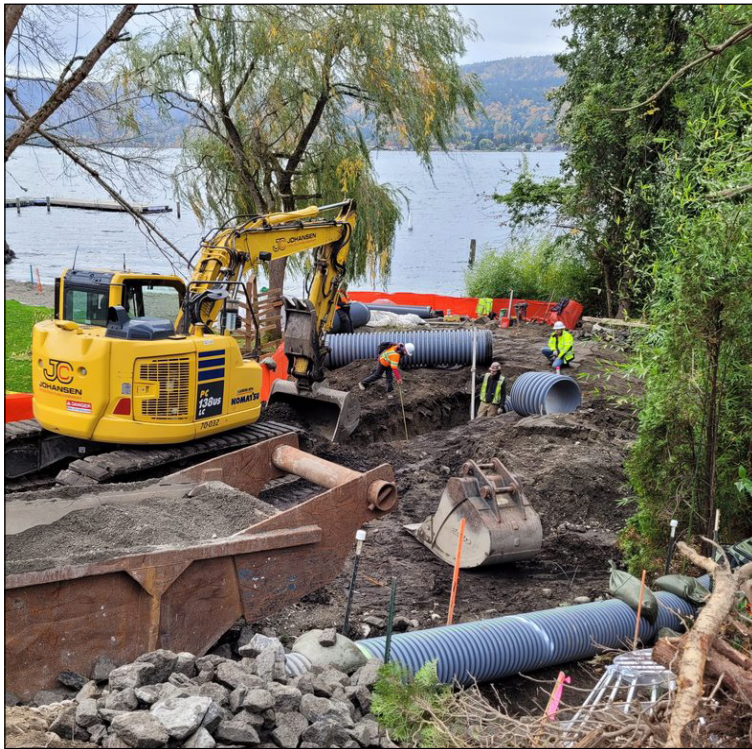
Excavating a drain line and installing drain pipe for a storm water outfall. A temporary storm water bypass runs through the pipe in the foreground.
