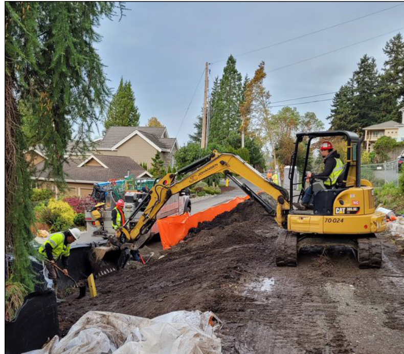
A crew widens the trail prism and begins excavating for a new retaining wall. The retaining wall will support the wider trail and its shoulders.
