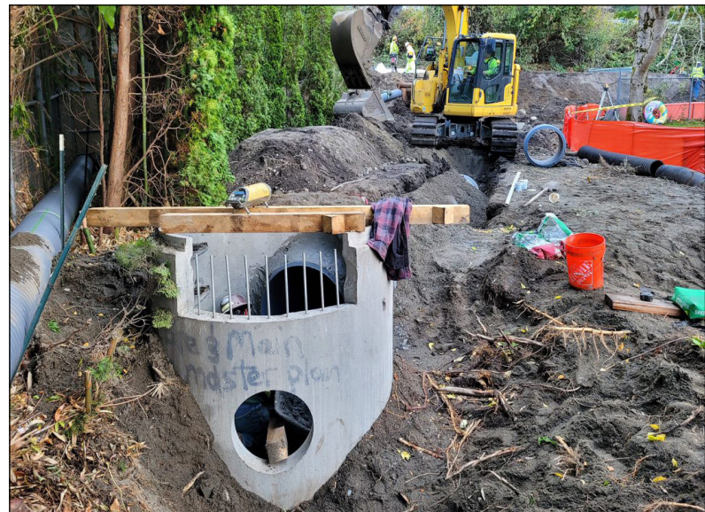
Installation in progress for the drainage outfall structure on the system in the two other photos on this page.
