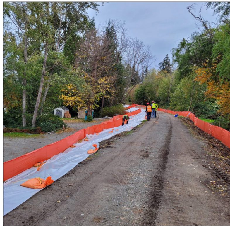
Preparing for rain, crews install plastic sheeting on exposed banks, and inspect the erosion control fence that will direct rainwater to existing outfalls.
