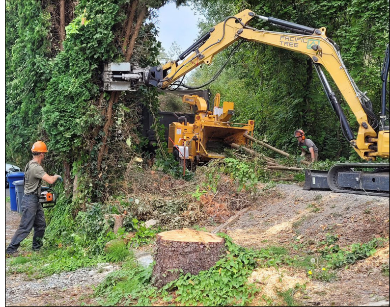
Crews remove and mulch trailside trees in the narrow space between the trail and adjacent street.
