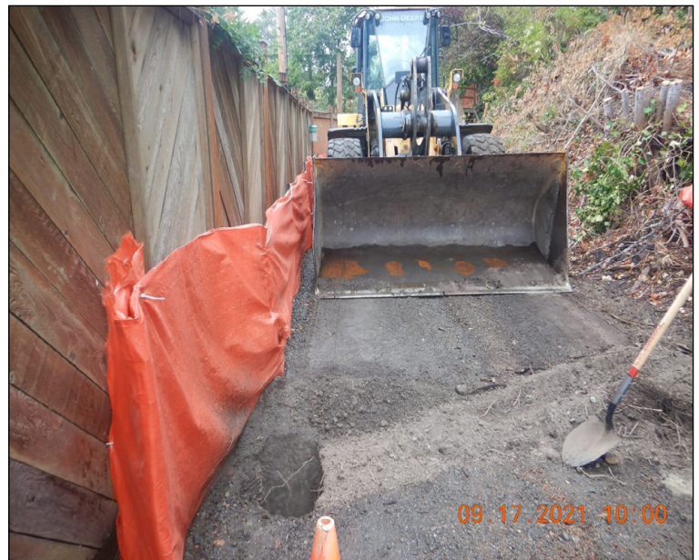
Locating buried utilities under the trail in close proximity to private home and fences.
