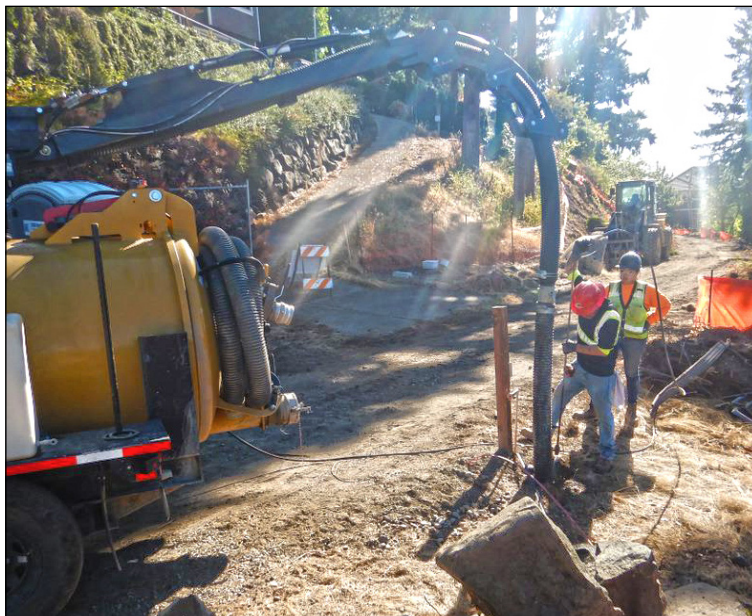
Crews use a vactor trailer to pothole, making a small diameter hole to uncover buried utilities.
