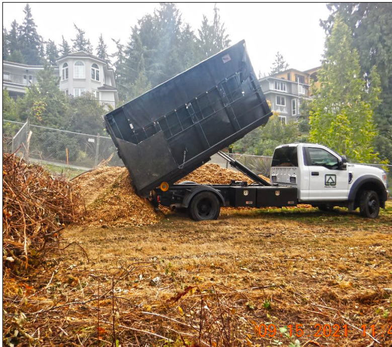
Wood mulch produced during trailside clearing is stockpiled for later use on the project.
