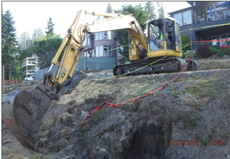
An excavator removes soil along the trail's edge to expose utility lines.
