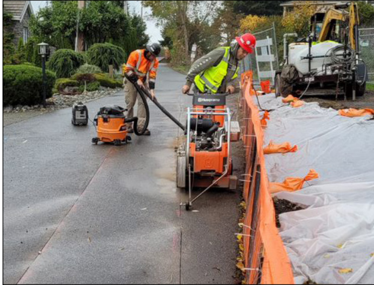
Roadway is saw cut before a section is removed to install a new drainage line, ensuring a precise cut in the asphalt.
