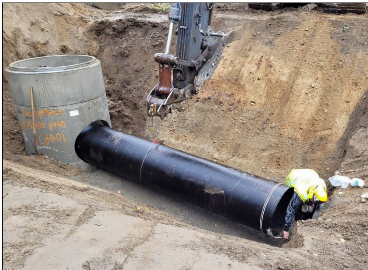
Once completed, this new storm drainage system will convey storm water off the trail.
