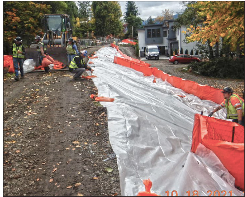
Crews improve trailside erosion control measures in preparation for wet weather.
