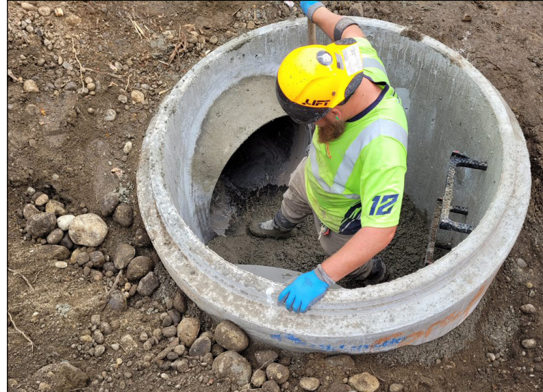
A team member inspects the joint between a newly installed catch basin and storm water drain pipe.
