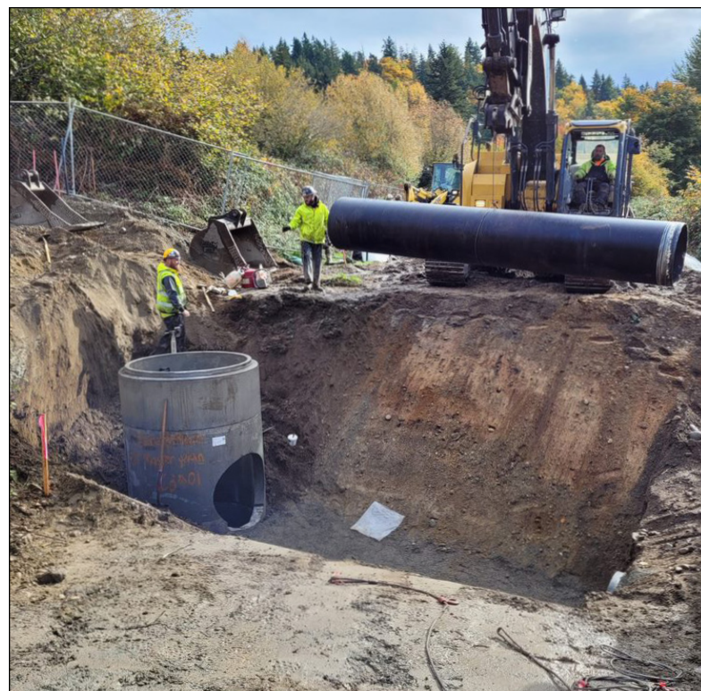
A new storm water drain pipe is lifted into position, where it will connect to the new concrete catch basin at left.
