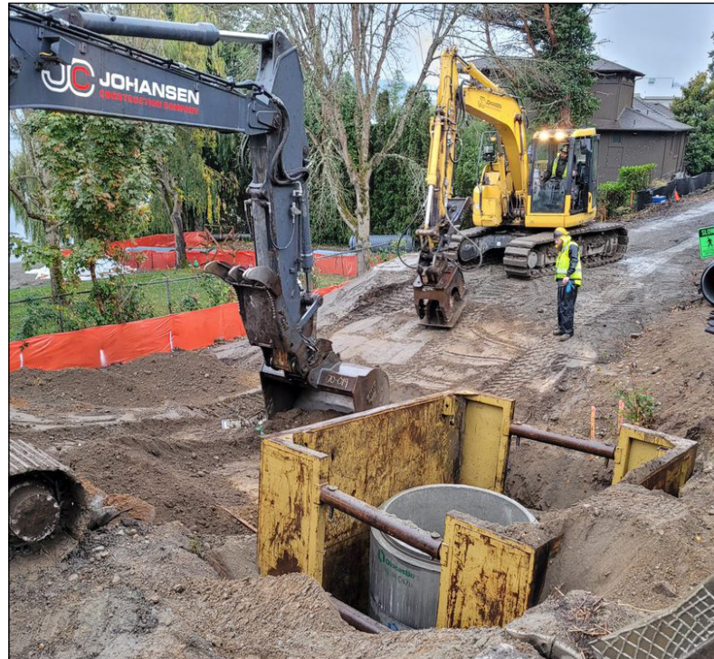
A shoring box protects the excavation around the new catch basin (foreground) while a crew removes a section of trail to install a connecting drain pipe.
