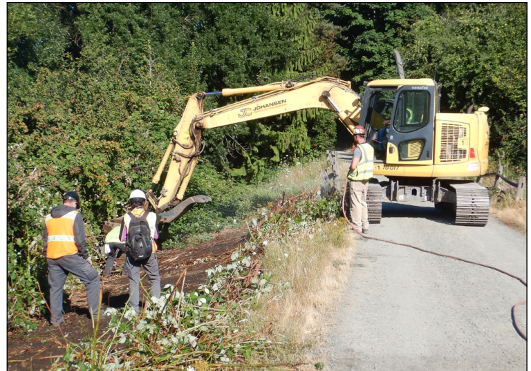
Removing brush before site and erosion control fence is installed.
