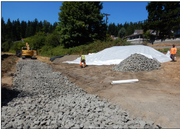
Building the construction vehicle entrance at SE 33rd Street.
