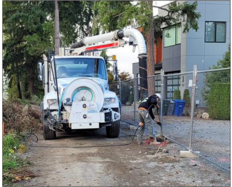
A vactor truck is used to remove soil above buried utility lines.
