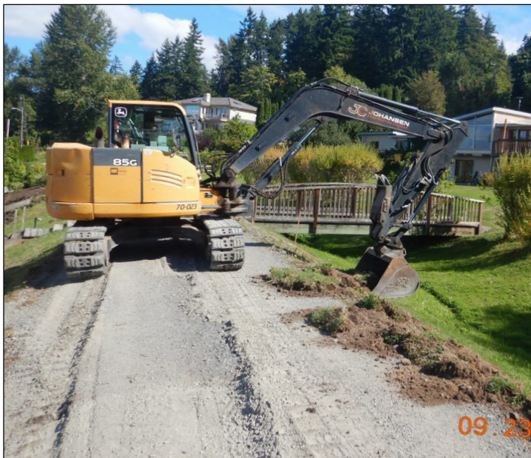
Removing grass and top soil to prepare trail footprint.
