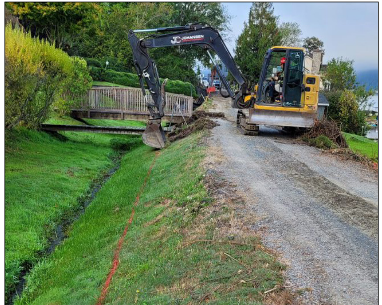
Removing grass and top soil to prepare trail footprint.
