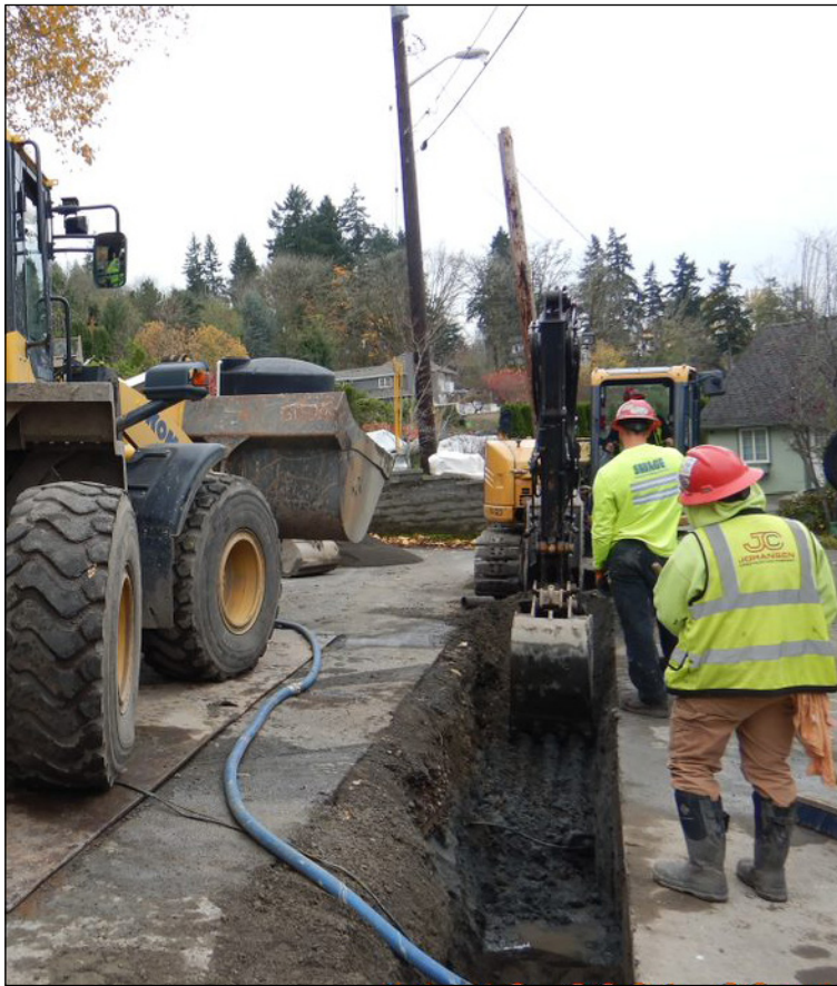
A crew uncovers an existing water main that will be moved to provide space for storm water drainage improvements.
