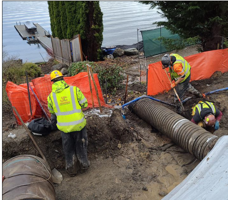
Team members prepare the area around an existing storm drainpipe for a new retaining wall. The wall (wall 5) will be built over and around the pipe.
