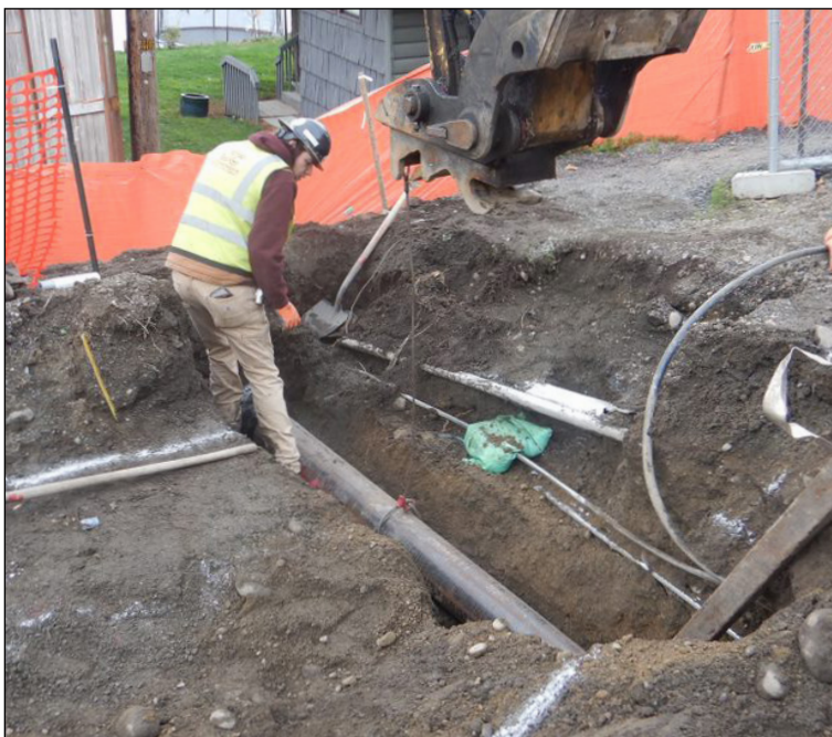
Crews relocate buried utility lines to facilitate new retaining wall (wall 5) construction.
