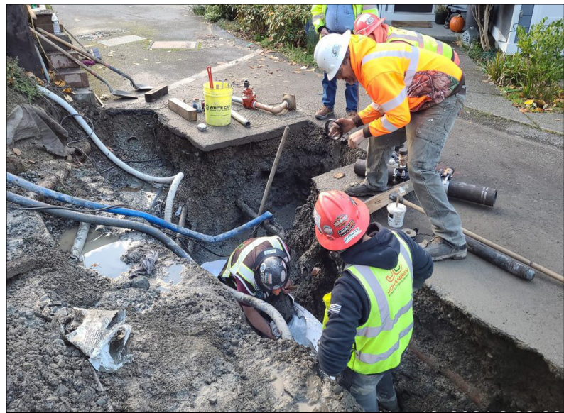
The crew installs new sections to an existing water main to route it around a planned drainage system.
