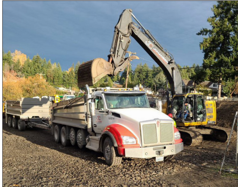
Loading soil excavated during retaining wall construction, to be removed from the project site.
