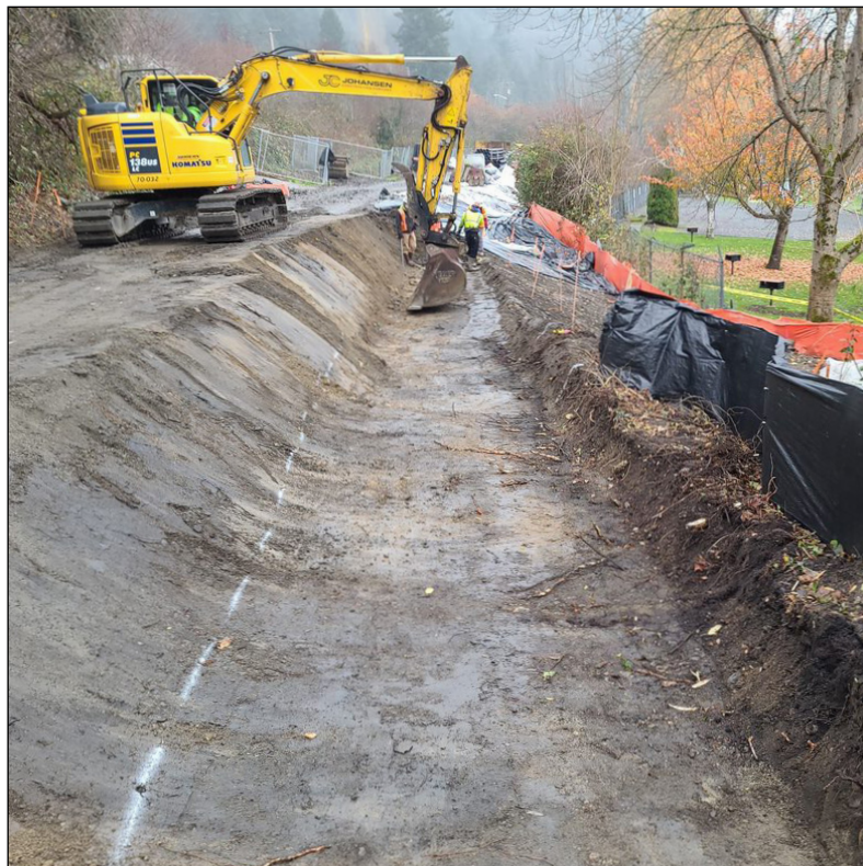
Making final inspections on the retaining wall (wall 1) excavation near SE 33rd Street, wall construction will begin soon.
