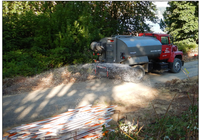
A water truck wets the trail surface to prevent dust from leaving the construction site.
