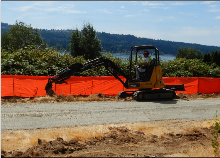
Clearing along the trail, inside of the erosion control fencing.
