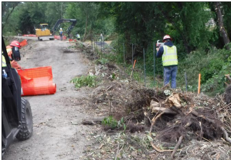
Crews install posts for high visibility fence near the edge of the trail construction boundary.
