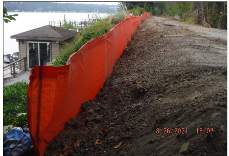
High visibility fence installed, with earth securing the fence bottom, to prevent erosion during trail construction.
