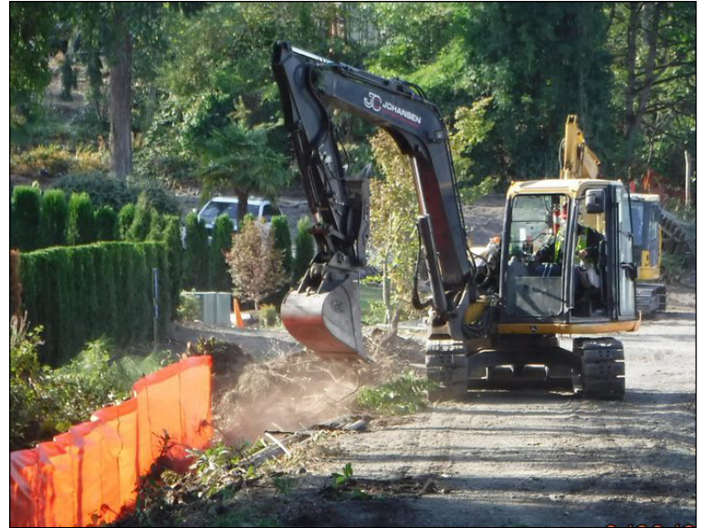
An excavator clears brush along the trail, and crews install high visibility silt fence immediately behind the excavator.
