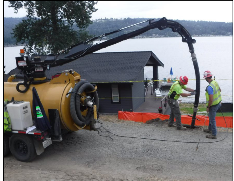
Crews use a vector trailer to excavate a small diameter “pothole” in order to locate a utility line under the trail.
