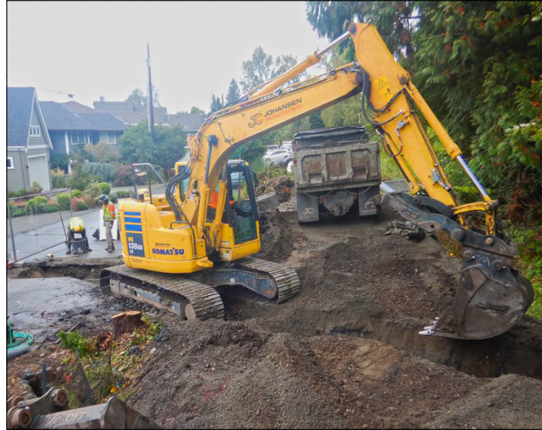
A excavator digs a channel for a new drainage system under the trail.
