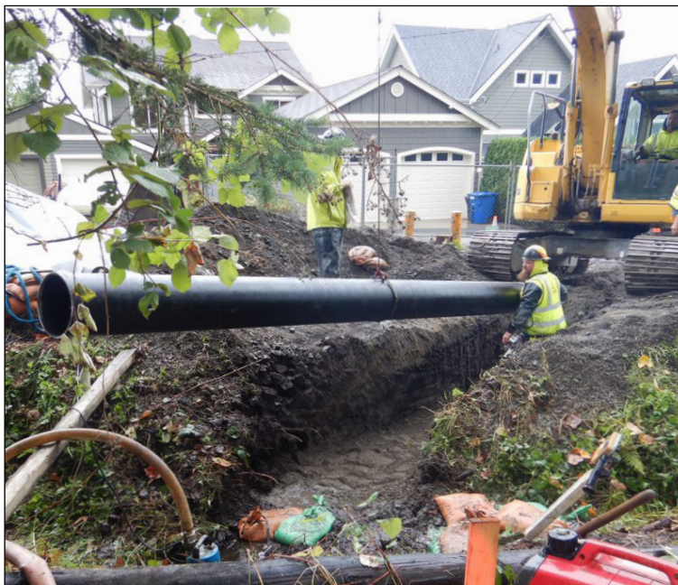
The first section of drainage pipe is lowered into the newly excavated channel.
