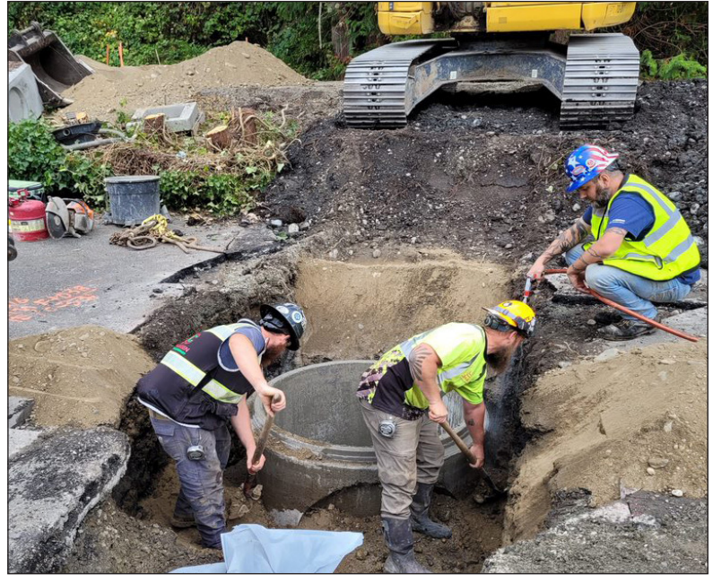
A catch basin is installed adjacent to the trail, and will be the junction between two new drain lines.
