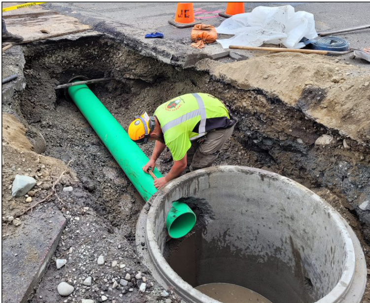
A new drain line is installed to connect the new drainage system to an existing drain pipe.
