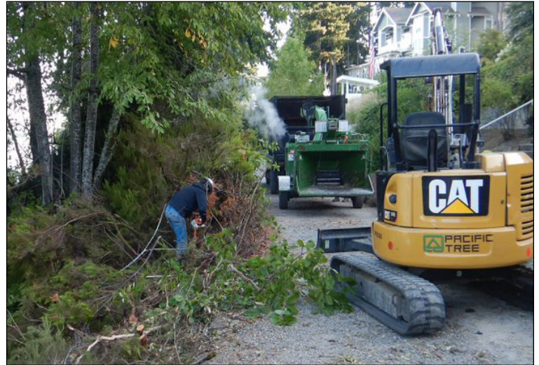
Trailside vegetation is cleared by hand and excavator, and converted to mulch onsite.
