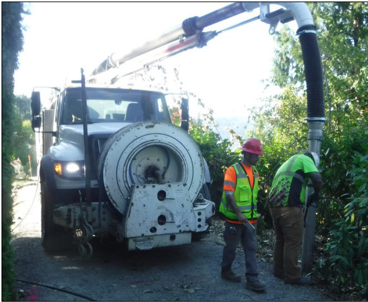
Potholing: Crews making a pothole diameter hole in the trail to locate a buried utility line.
