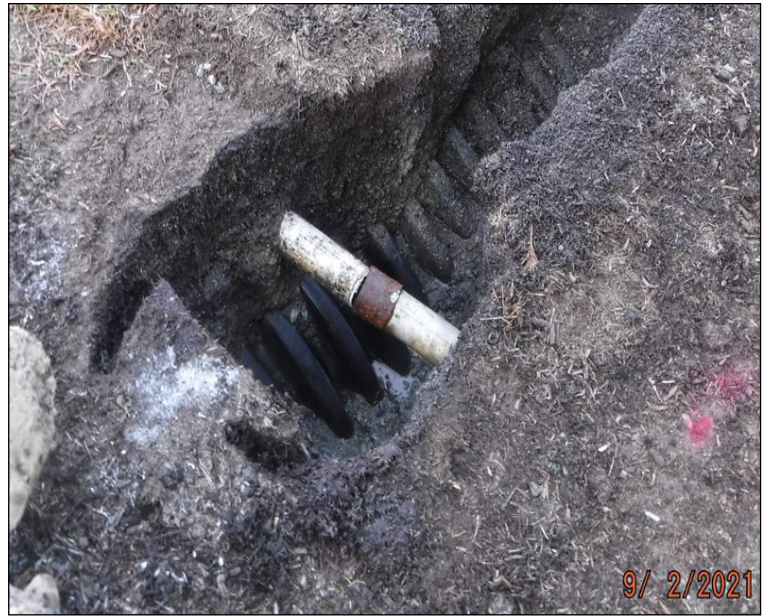
The result of potholing: a buried line is found ahead of future trail work.
