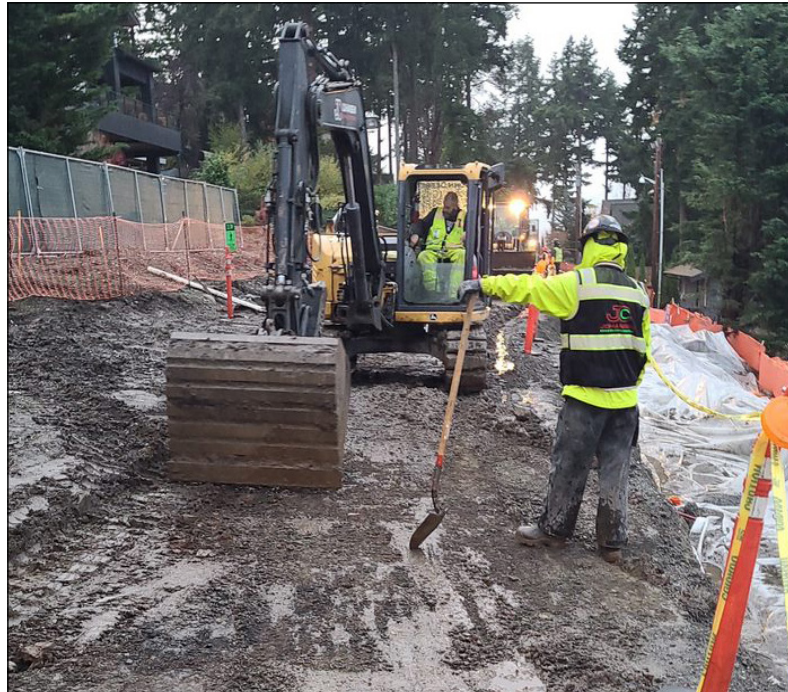
Crews worked on wall #5, a 354-foot retaining wall, this week. Here preparing to add gravel to the trail adjacent to the wall site.
