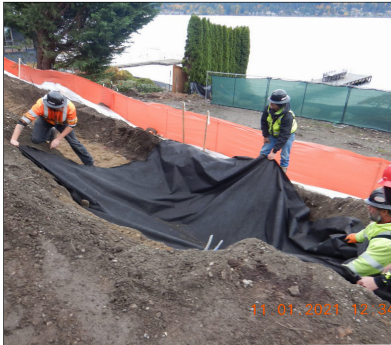
Crews install geotextile at the bottom of the excavation to separate the soil beneath from gravel to be installed next.
