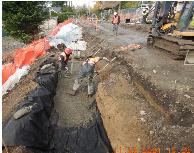
Crews backfill the excavation with gravel, which once compacted will provide a stable base for the wall's footing.
