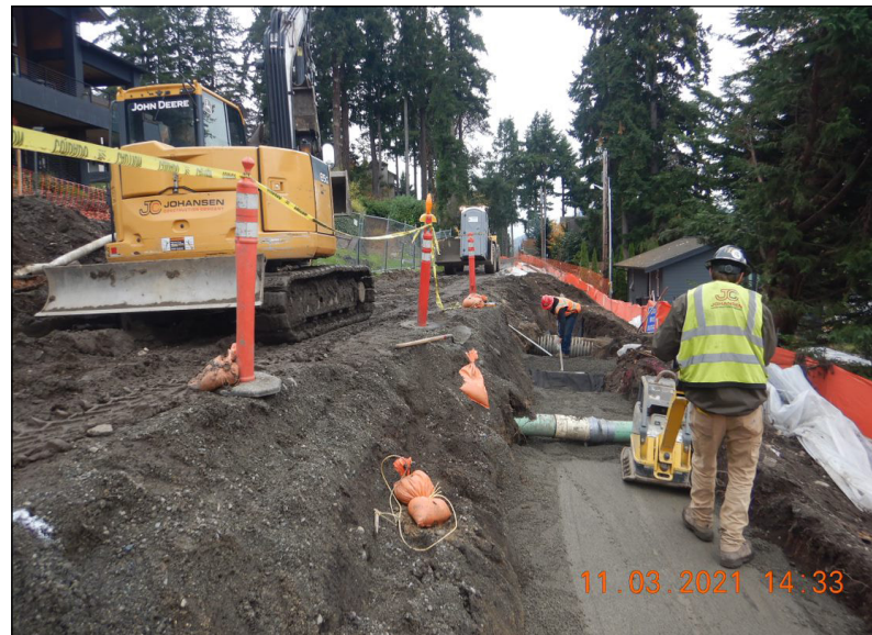
The gravel base is compacted in the foreground, while a team member rakes in gravel around an existing utility line.
