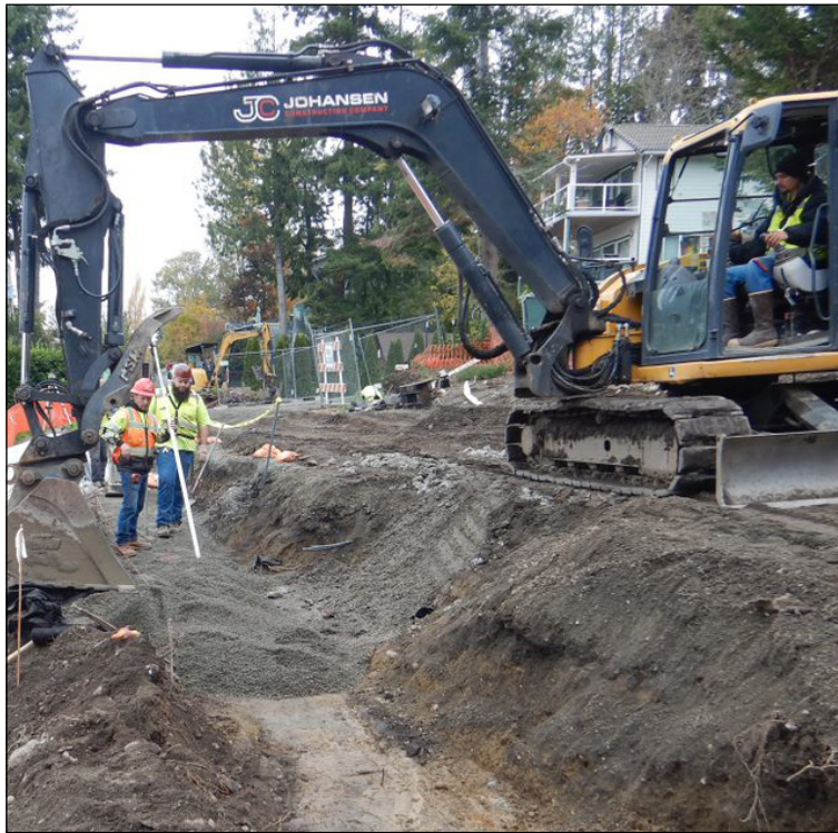
Crews spread the retaining wall's gravel base, carefully checking the depth to ensure the retaining wall's finished elevation will be correct.
