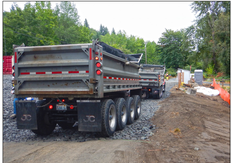
Trucks depart the site over the stabilized construction entrance, which is created to reduce the amount of sediment transported onto paved roads by vehicles.
