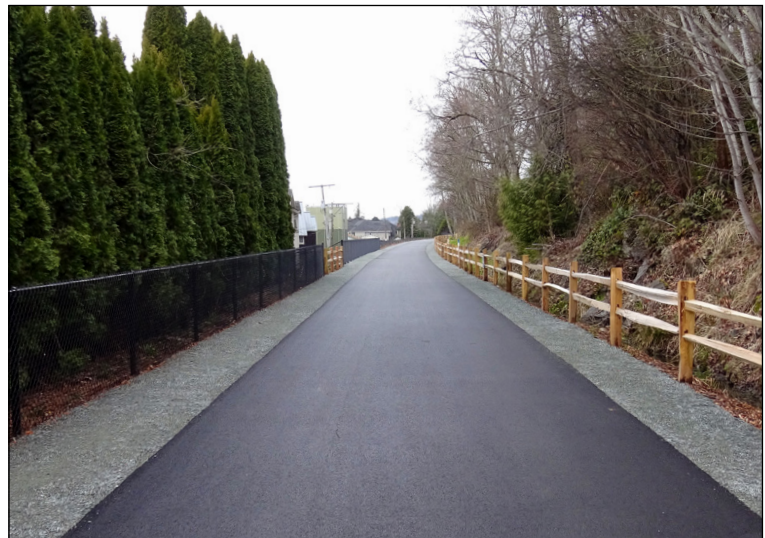
...with a 12-foot wide paved trail and 2-foot gravel shoulders, landscaping, and other trail amenities.
