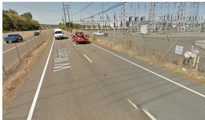
Photograph 3. West Marginal Place South at the southern edge of the Seattle City Light facility, facing northwest.
