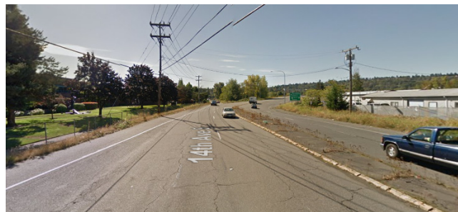
Photograph 4. 14th Avenue South at the South Director Street intersection, facing south.
