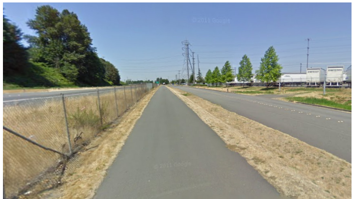
Photograph 1. The Green River Trail and 27th Avenue South at the edge of Cecil Moses Park, facing northwest.
