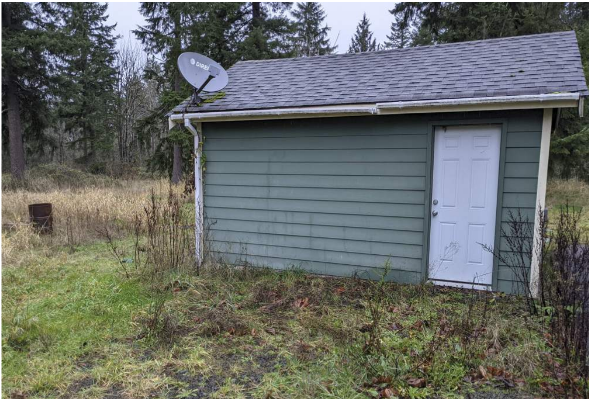
Figure 6: Photo of building labeled "Existing Well house" on survey.
